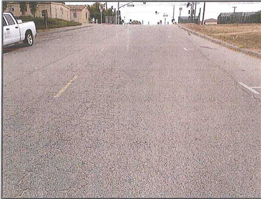
MONTEREY COUNTY JAIL FACILITY PHOTO NO. 5 - NATIVIDAD ROAD TO PERIMETER DRIVE
