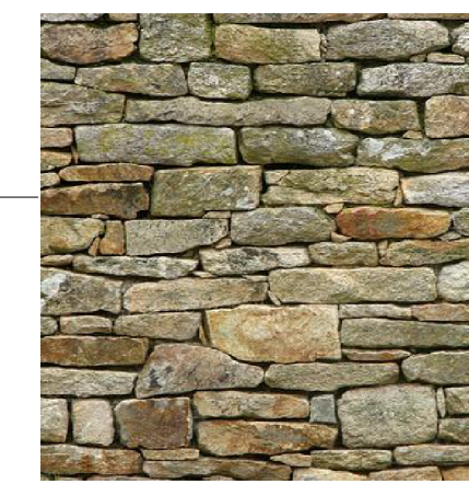
STONE CLAD RETAINING WALL
