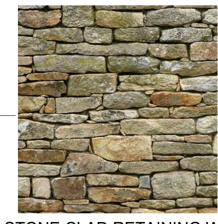
STONE CLAD RETAINING WALL
