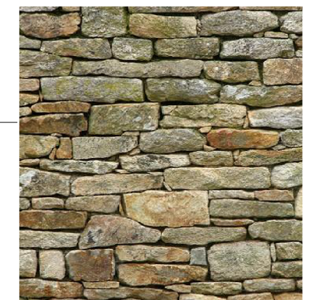
STONE CLAD RETAINING WALL
