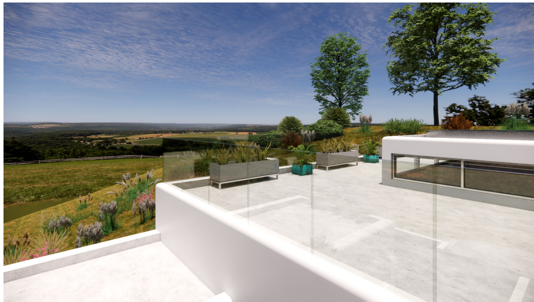
SEAMLESS GLASS RAILING ANCHORED IN PARAPET
