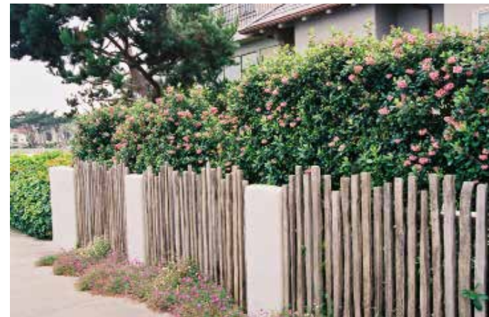
Rustic stucco screen fence
