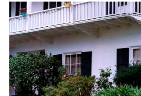
Exposed rafter tails add character to Mediterranean Revival eaves.
