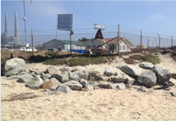
Rip rap in front of the MLML Shorelab
