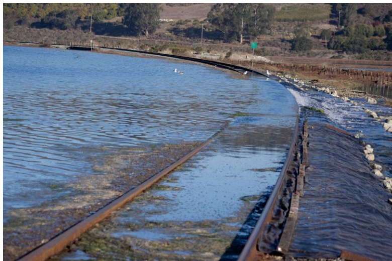
Image 3. Jan 1, 2014 King Tide pours over the railroad tracks between Kirby Park and the Elkhorn Research Reserve (Photo: Fred Hochstaedter)
