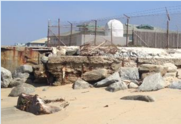
Remnant concrete structure in front of MLML Shorelab
