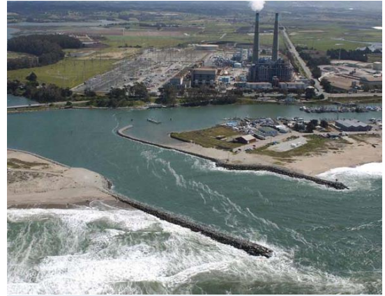
Figure 4. Moss Landing Harbor levees (Coastal Records Project, Kenneth & Gabrielle Adelman)
