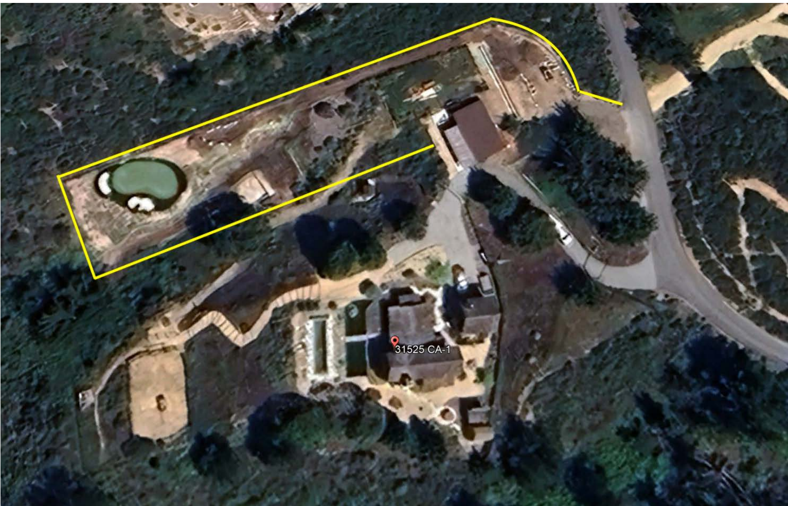
Figure 1. Area of concern that was impacted by non-permitted grading activities is located within yellow rectangular shaped area.
