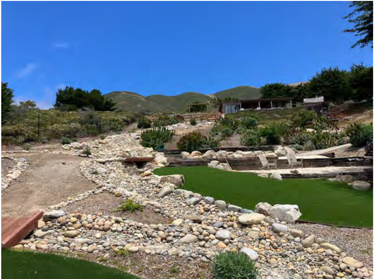
Figure 3. View of putting green area consisting of artificial turf and rock drainage swale that was constructed.
