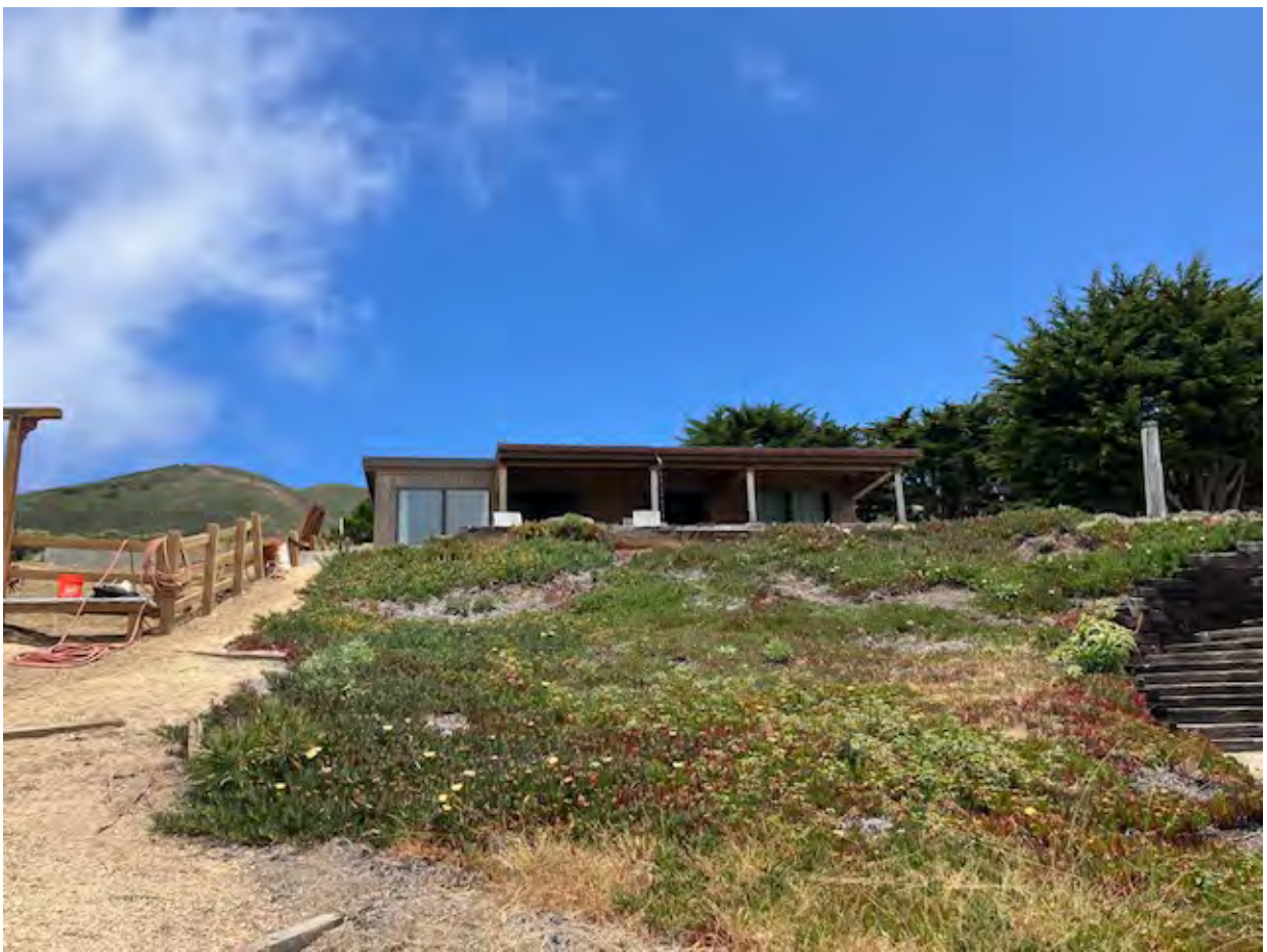
Figure 10. ADU/guesthouse is located upslope of the putting green and rock drainage swale area. Exotic ice plant is common at the site.
