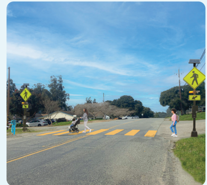
Rectangular Rapid Flashing Beacons at the crosswalk near Prunedale Elementary School
