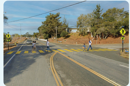
Rectangular Rapid Flashing Beacons at the crosswalk on Hall Road at Sill Road
