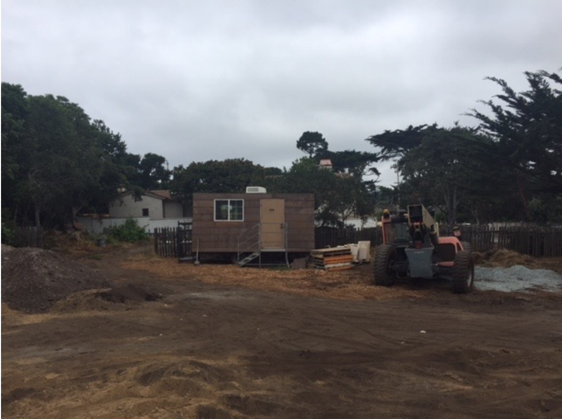
Figure 2. Another view of disturbed and impacted property. The neighboring property at 26338 Valley View is located on other side of trailer and small fence
