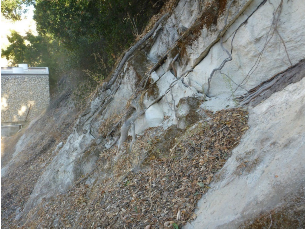
2019 Photograph 7. Roots growing along bedding planes dipping out of slope in outcrop upstream of Powerhouse and exposed penstock.
