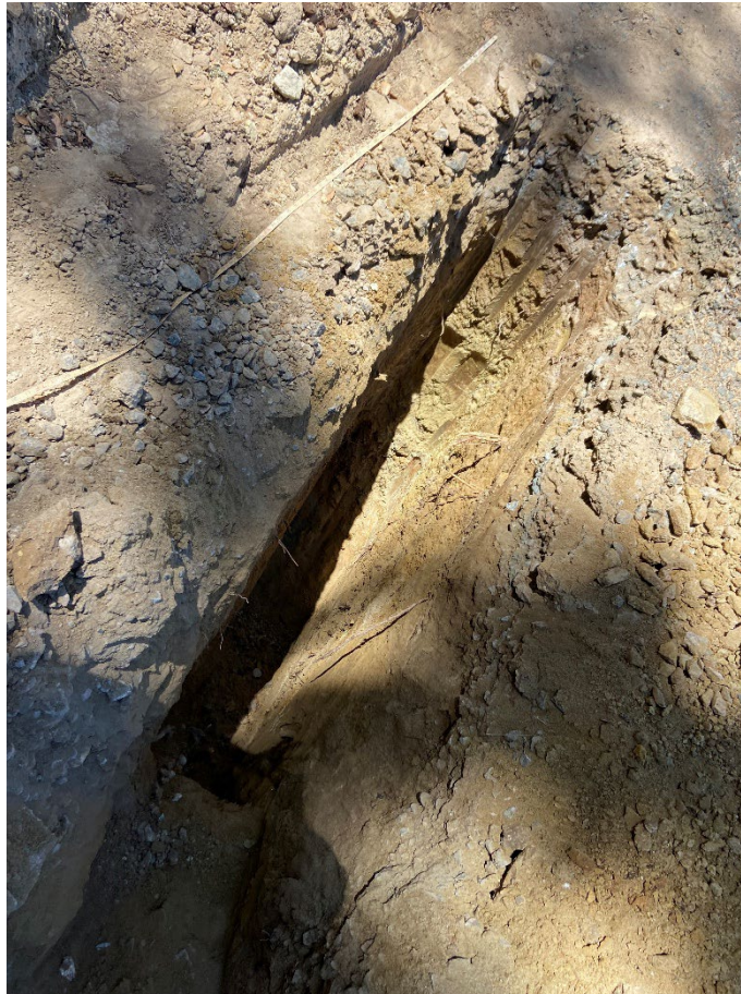
Photo #4: Excavation of TP-2, Downhole
