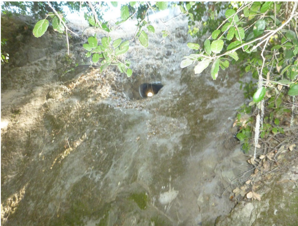
2019 Photograph 20. Culvert beneath Lake Nacimiento Drive. Note the culvert appears partially collapsed but is open.
