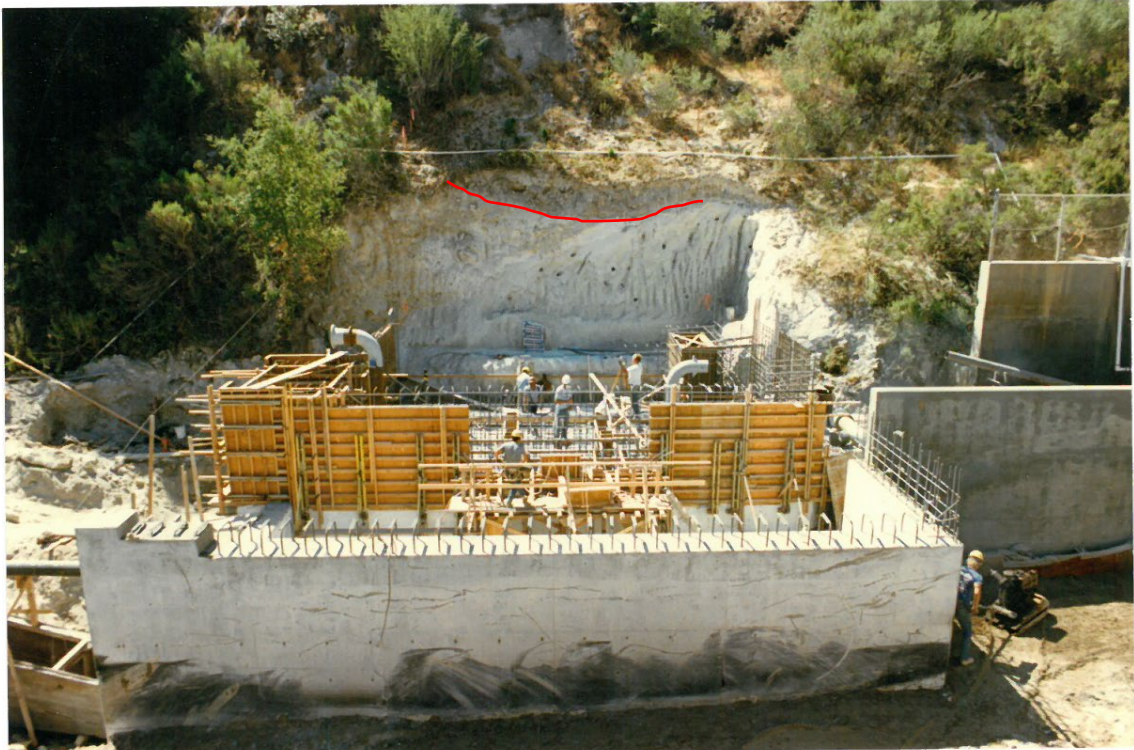
1986 Photograph 4. Powerhouse construction photograph (circa 1986) showing cut slope and debris-filled swale (above red line).
