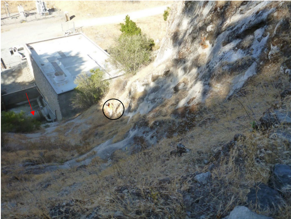
2019 Photograph 2. Looking down debris flow swale from access road. Note exposed penstock in middle left (arrow) and geologist (circled) for scale.
