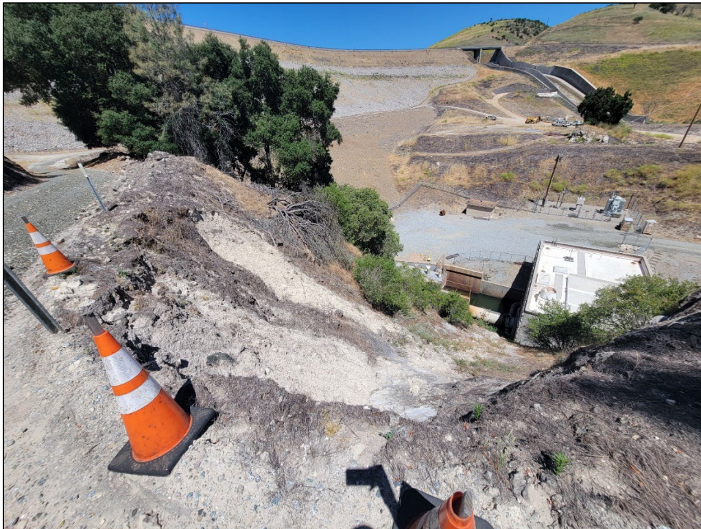
Photograph 2024-3. View of recent shallow failure above Powerhouse, and erosion along edge of access road. View is to the North.
