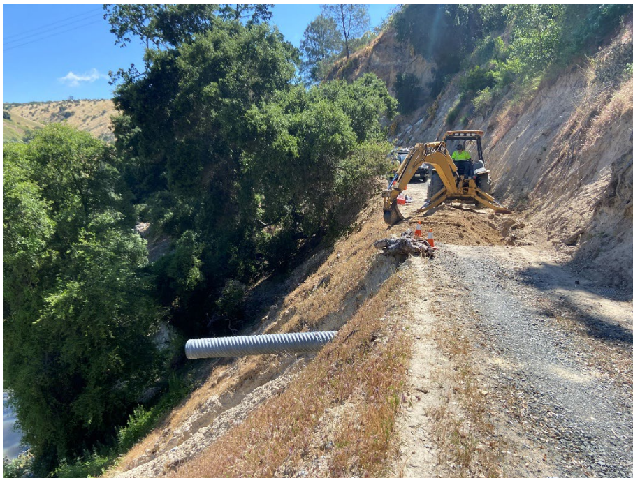
Photo #1: Excavation of TP-1, Looking East
