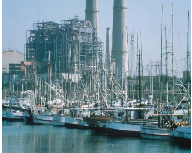
Figure HDD-1 – Moss Landing Harbor
