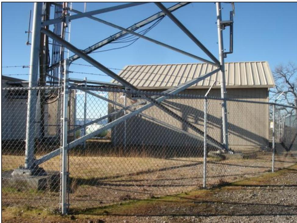
Photo 12: Chain link fence is not grounded
