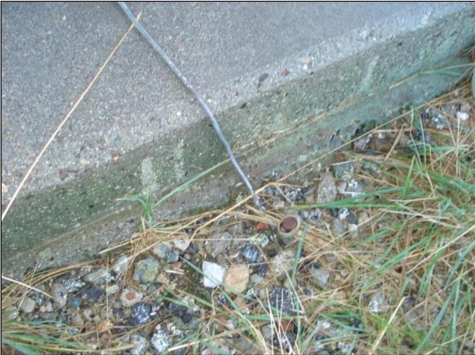
Photo 1: Individual ground rod installed at the tower leg
