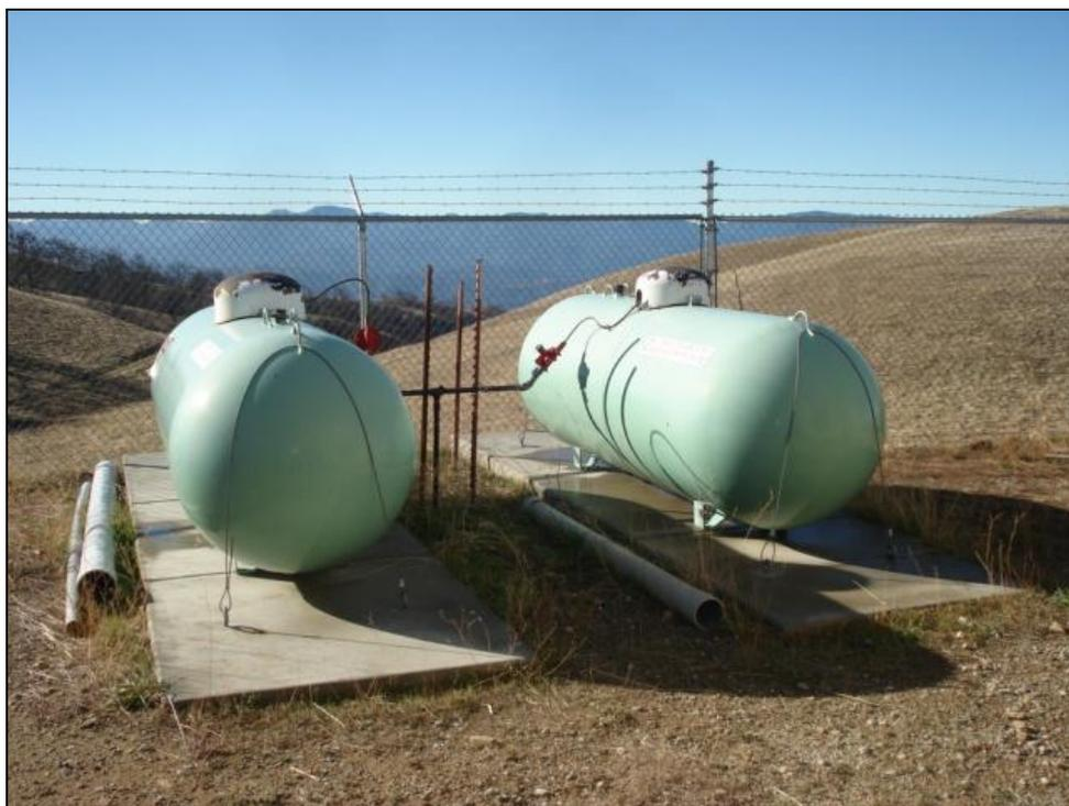
Photo 10: Fuel tanks are not grounded
