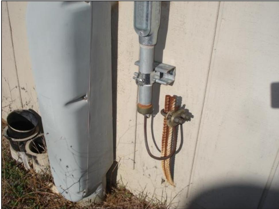
Photo 15: Panel "B" is grounded to the re-bar
