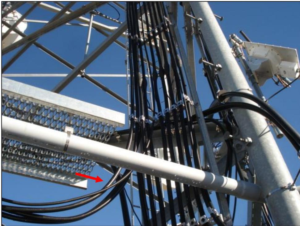
Photo 7: Coaxial cables turning into the shelter without grounding kits installed
