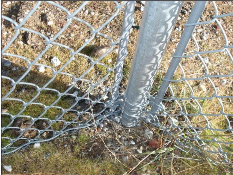
Photo 13: Fence post and gatepost are not grounded
