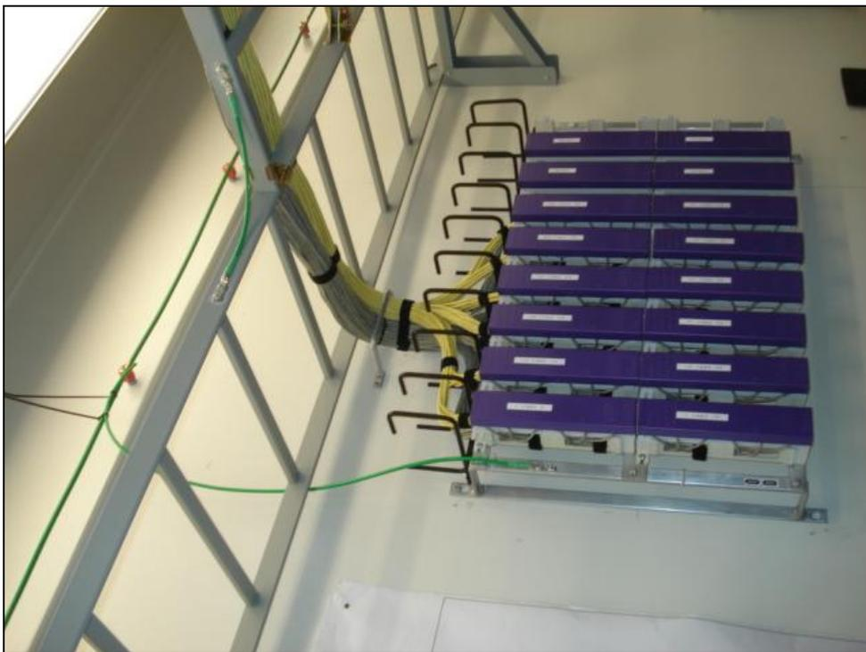
Photo 20: Telco is bonded to the Halo conductor
