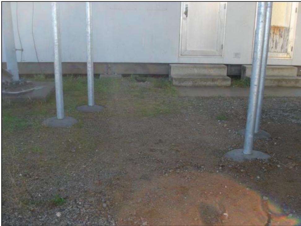
Photo 9: Ice-bridge support posts are not grounded
