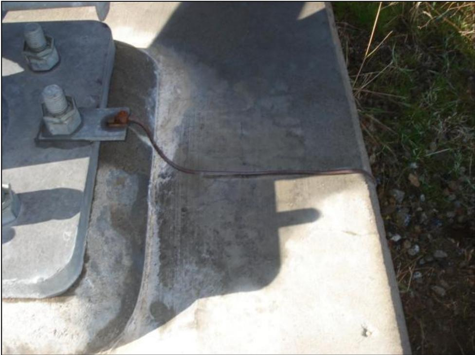
Photo 2: Tower leg grounding connection
