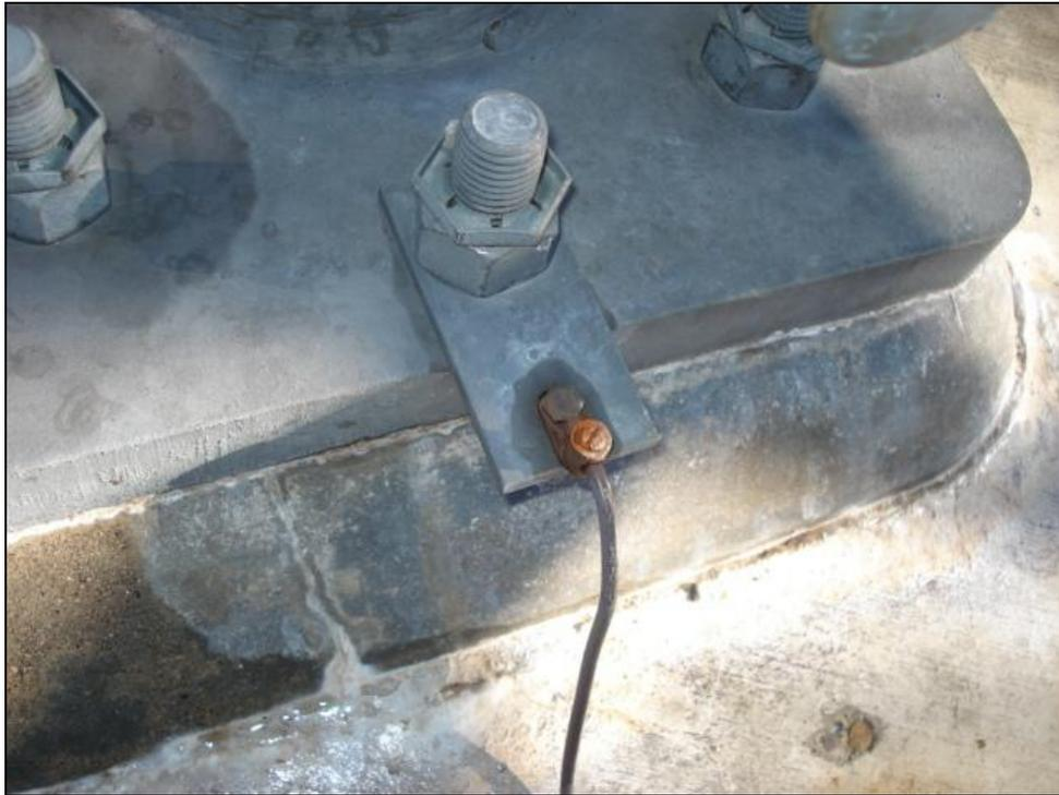
Photo 3: The connection appears corroded
