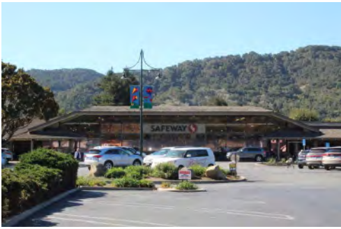
① Building A - Safeway
