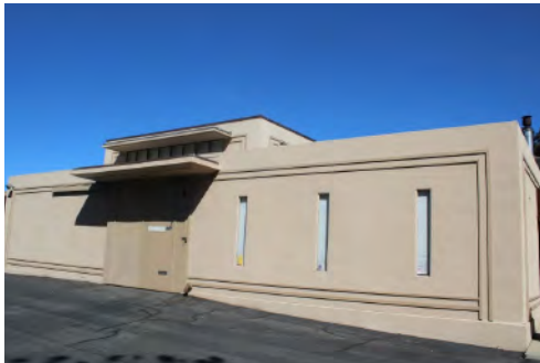
② Building B
