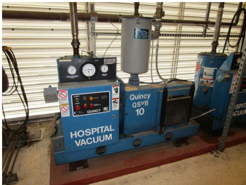
Medical vacuum systems are at the end of their expected useful lives.
