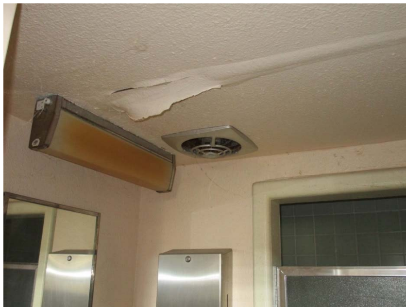
Ceiling exhaust fan is at the end of its expected useful life.
