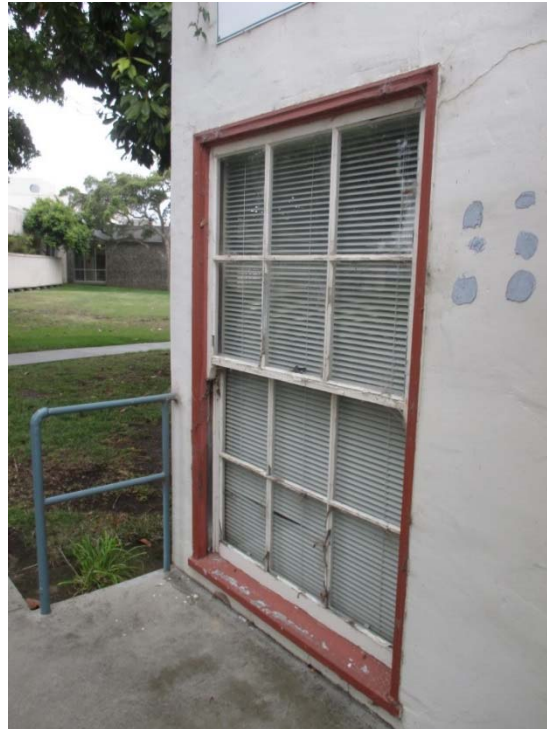
Exterior windows are ready for replacement
