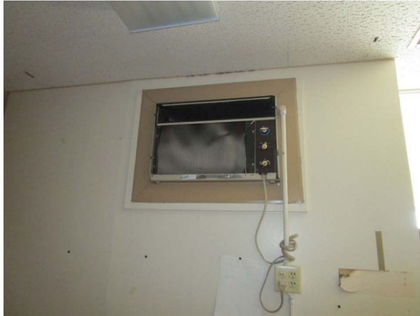
Wall mounted AC unit is at the end of its expected useful life.
