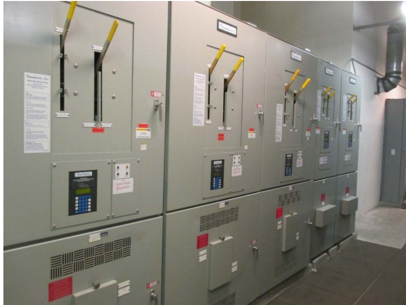
The automatic transfer switches have reached the end of their expected useful lives.
