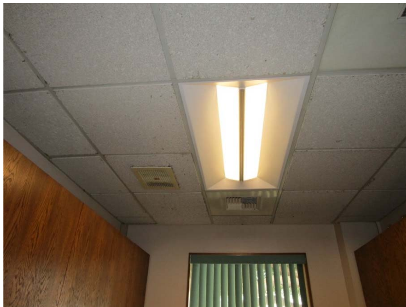
Ceiling exhaust fan is at the end of its expected useful life.
