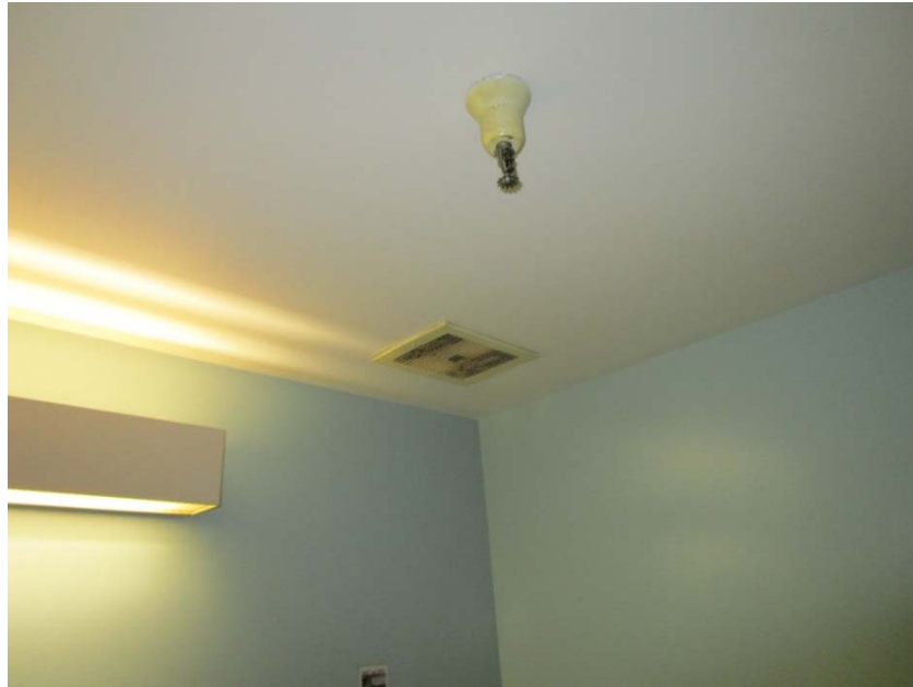
Ceiling exhaust fan is at the end of its expected useful life.
