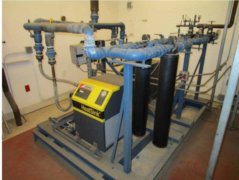
Refrigerated air dryer systems are at the end of their expected useful lives.
