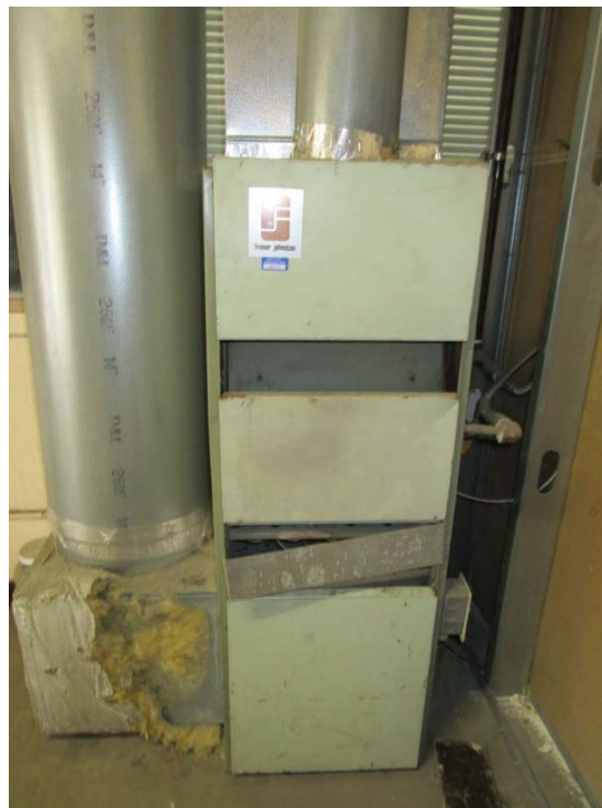
Gas furnace unit is at the end of its expected useful life.
