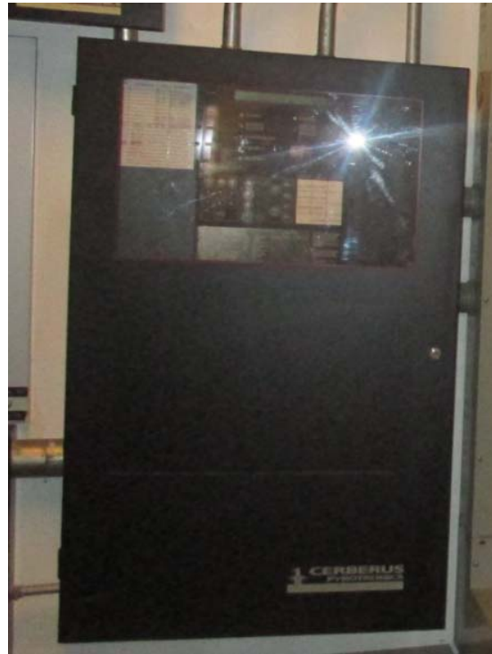
The fire alarm has reached the end of their expected useful lives.
