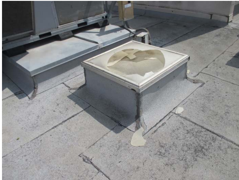
Damaged skylight
