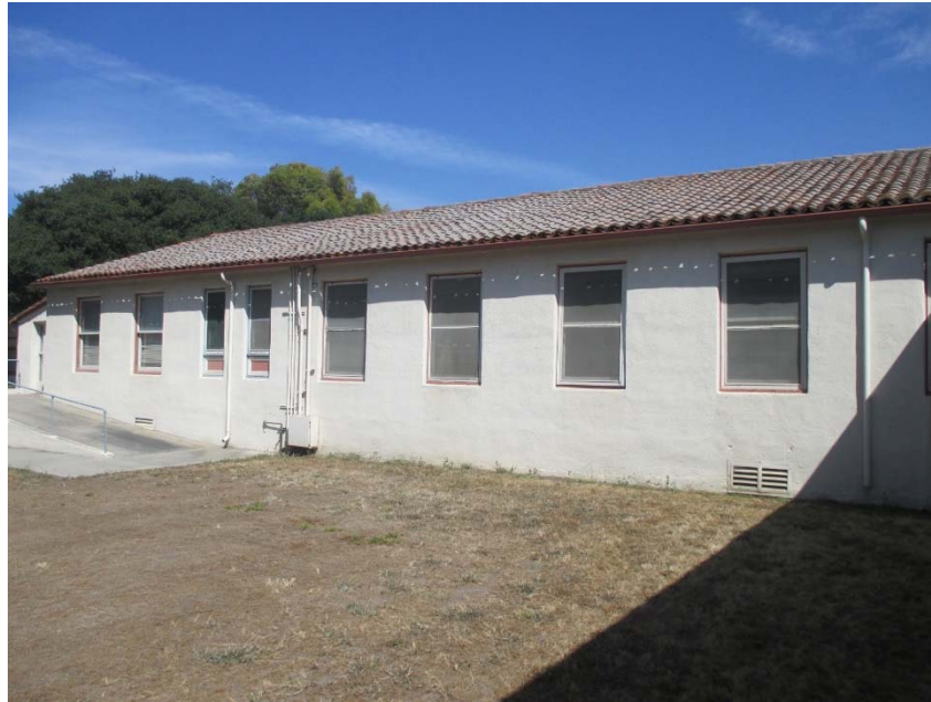
Exterior photo showing roof, wall finish and windows
