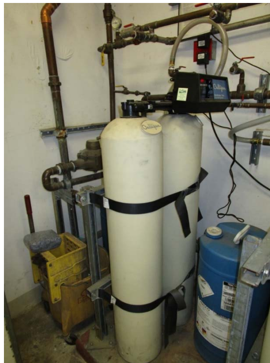
Water softener system is at the end of its expected useful life.
