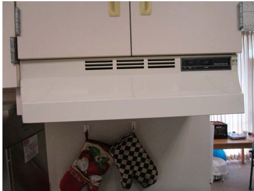
The range hood for the oven/range is at the end of its expected useful life.
