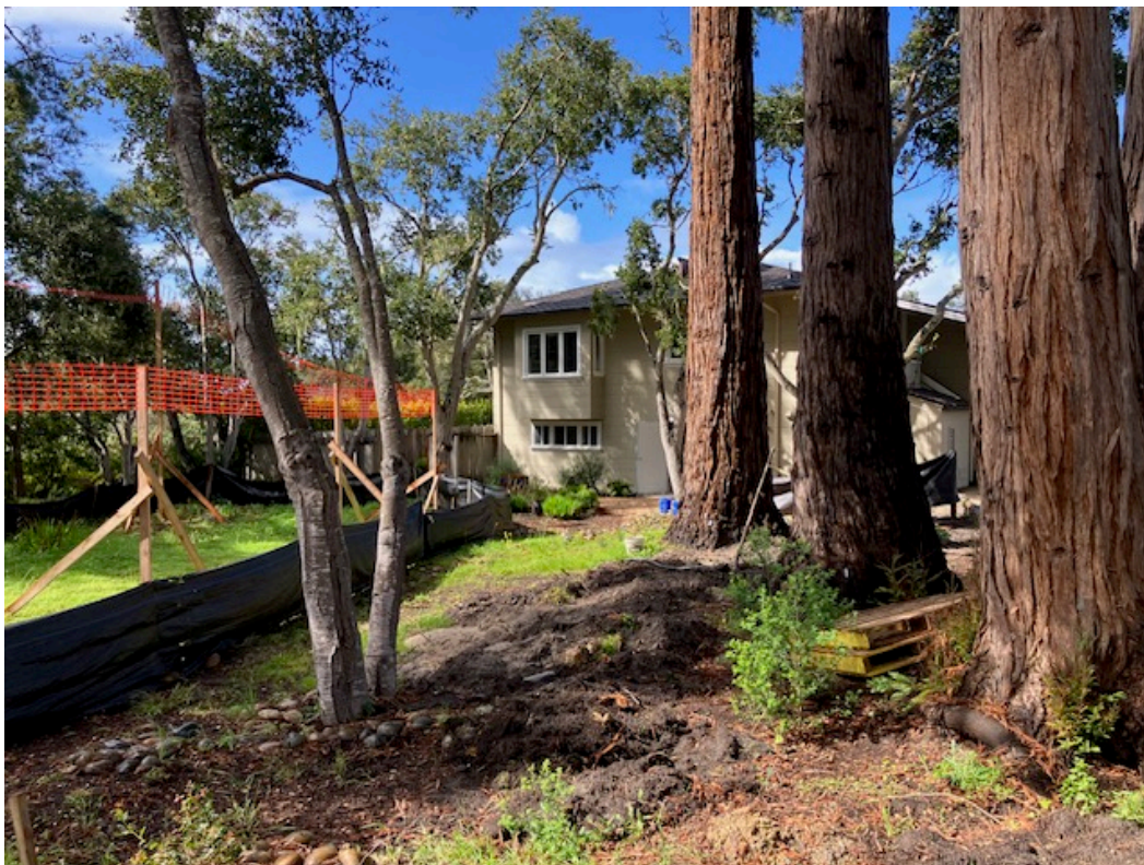
Figure 2. The ADU located a safe distance to the left of the redwoods will have a floated foundation to avoid and minimize root system impacts.
