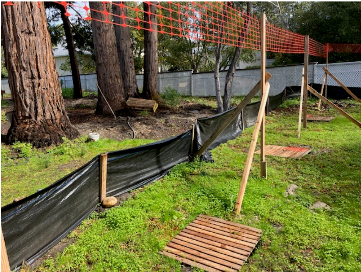
Figure 4. Three wood covers seen from lower center to upper right corner of photo identify the location of footings for the floated foundation.
