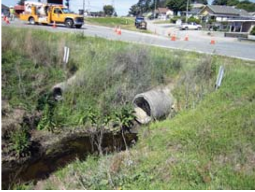
① Outlet of culverts under Las Lomas Drive to drainage channel along Hall Road
