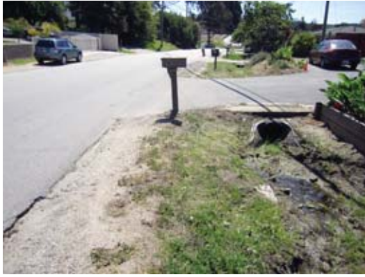
① Unlined drainage ditch parallel to Las Lomas Drive, adjacent to residential uses
