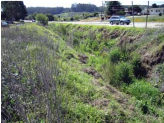
② Unlined portion of drainage channel, east from intersection of Hall Road and Las Lomas Drive
