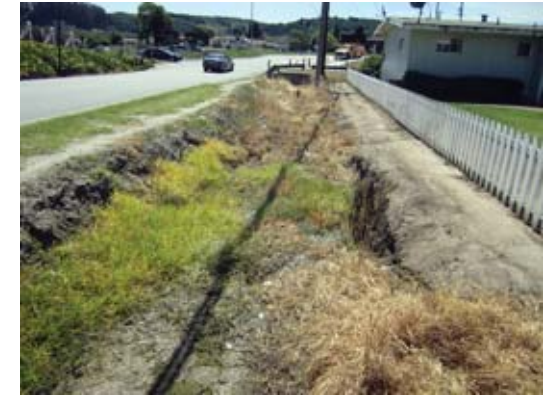
④ Unlined drainage ditch north of intersection of Las Lomas Drive and Hall Road, prior to entering culvert to drainage channel
