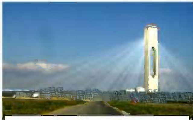
Figure 8: Seville solar power facility ( http://inhabitat.com/sevilles-solar-power-tower )
