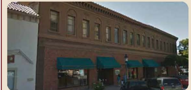
Vacant space on the 2nd floor of the Dick Bruhn building on Main Street could be redeveloped without providing any parking spaces.
