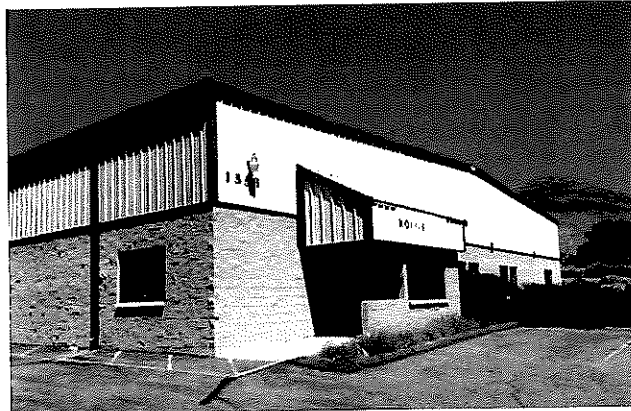
The Western Regional Facility.
