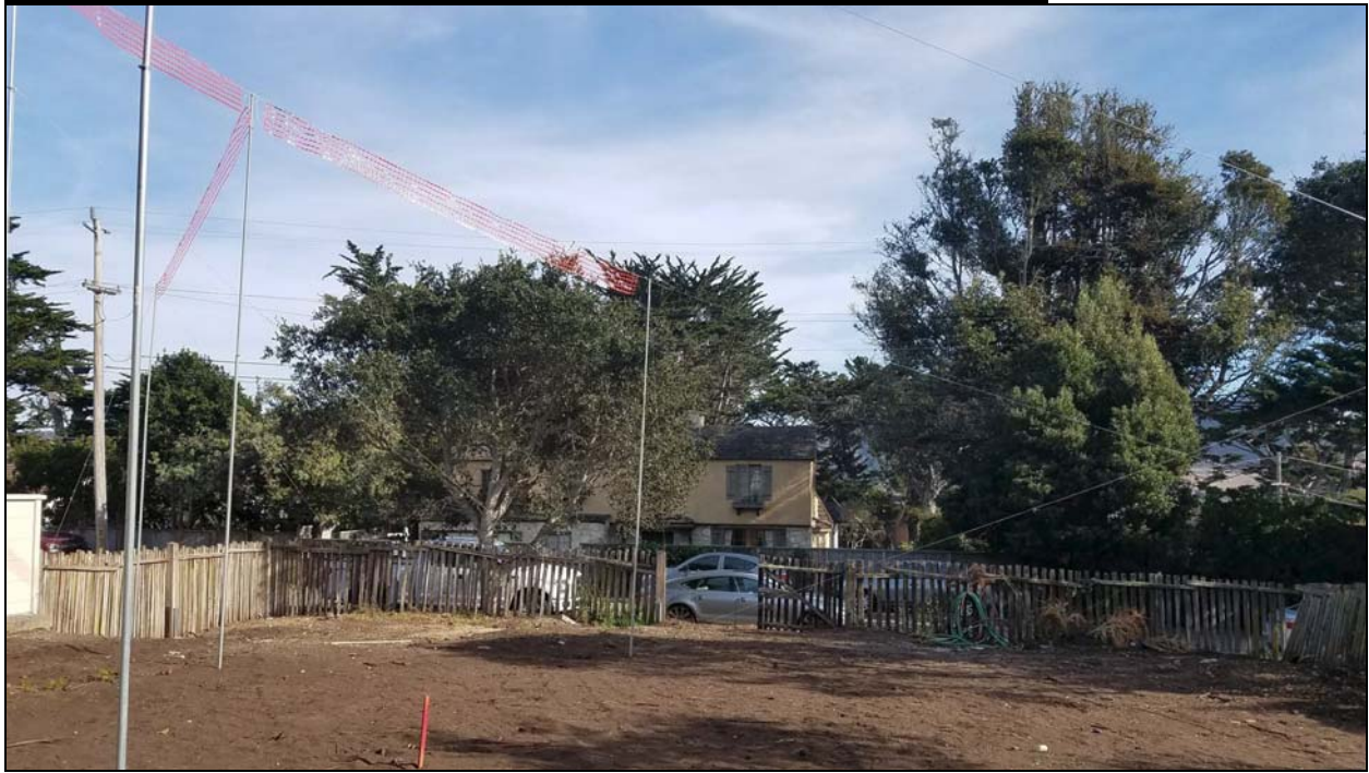
Figure 10a-14a – Site Visit Photos: Staking and Flagging (east) at 26346338 Valley View Avenue
