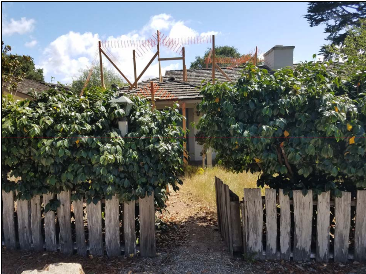
Figure 8a12a – Site Visit Photos: Staking and Flagging at 26346-338 Valley View Avenue g (west)
