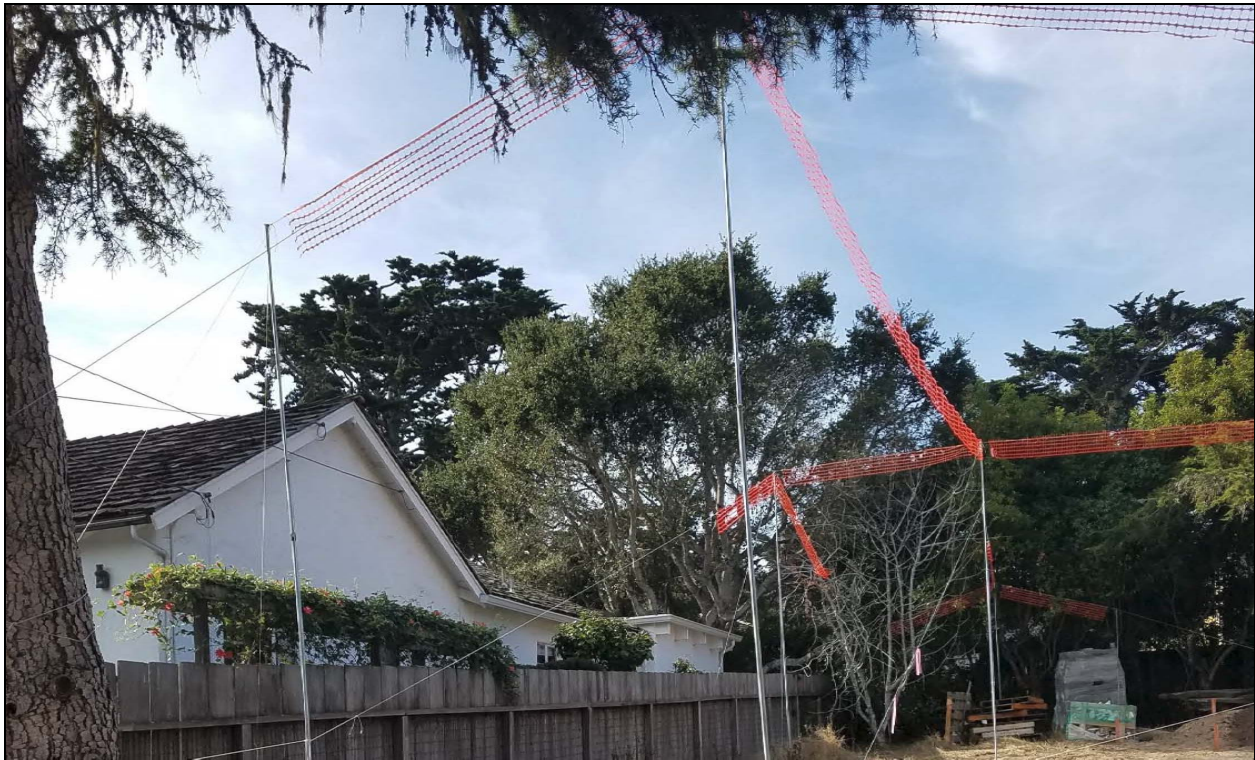
Figure 913b – Site Visit Photos: Staking and Flagging at 26338346 Valley View Avenue
