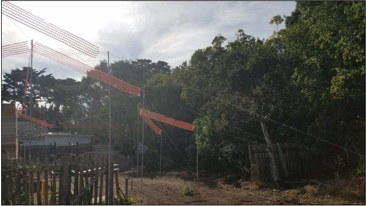
Figure 1014b – Site Visit Photos: Staking and Flagging at 2633846 Valley View Avenue
