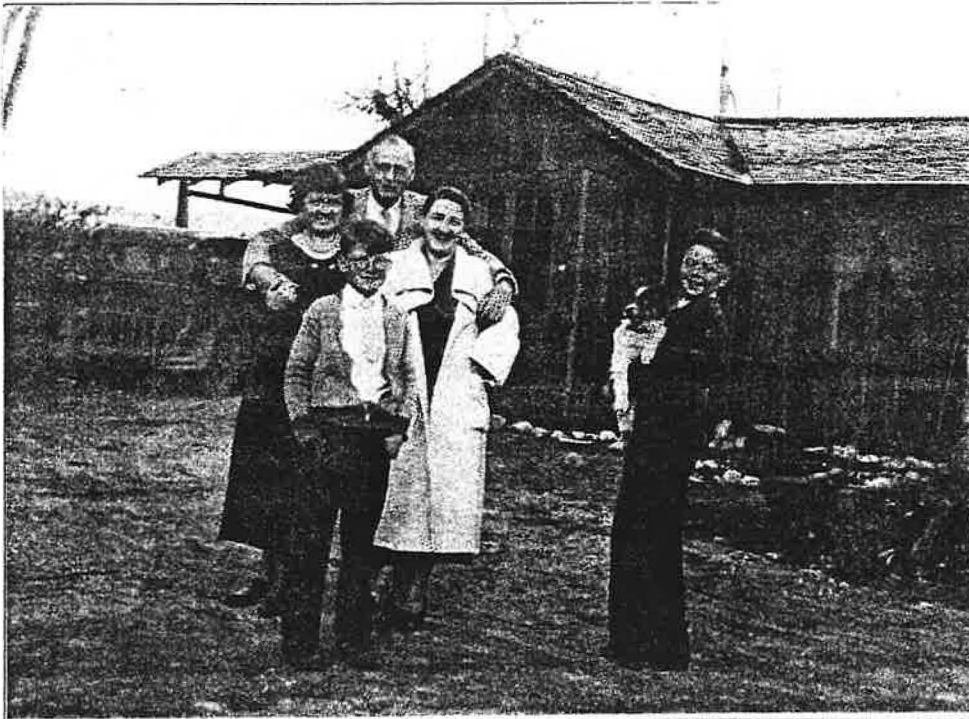
Description of Photo: (View, date, accession#) Looking NE at the w/facing facade of cabin #11, Orville Jones, 1934, Kathleen Jones Col., Phoenix, AZ
