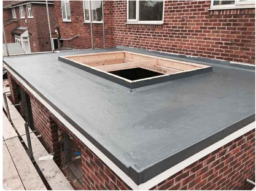
BUILT UP ROOF SYSTEM WITH HIGH ALBEDO / HIGH EMISSIVITY
