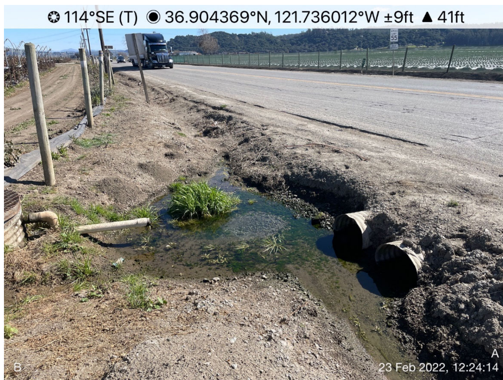
Photo 6. Inlet side of double 22"x12" CMP culvert crossing San Juan Road at Allison Street. These CMP pipes have a capacity of approximately 12 cfs prior to road overtopping.
