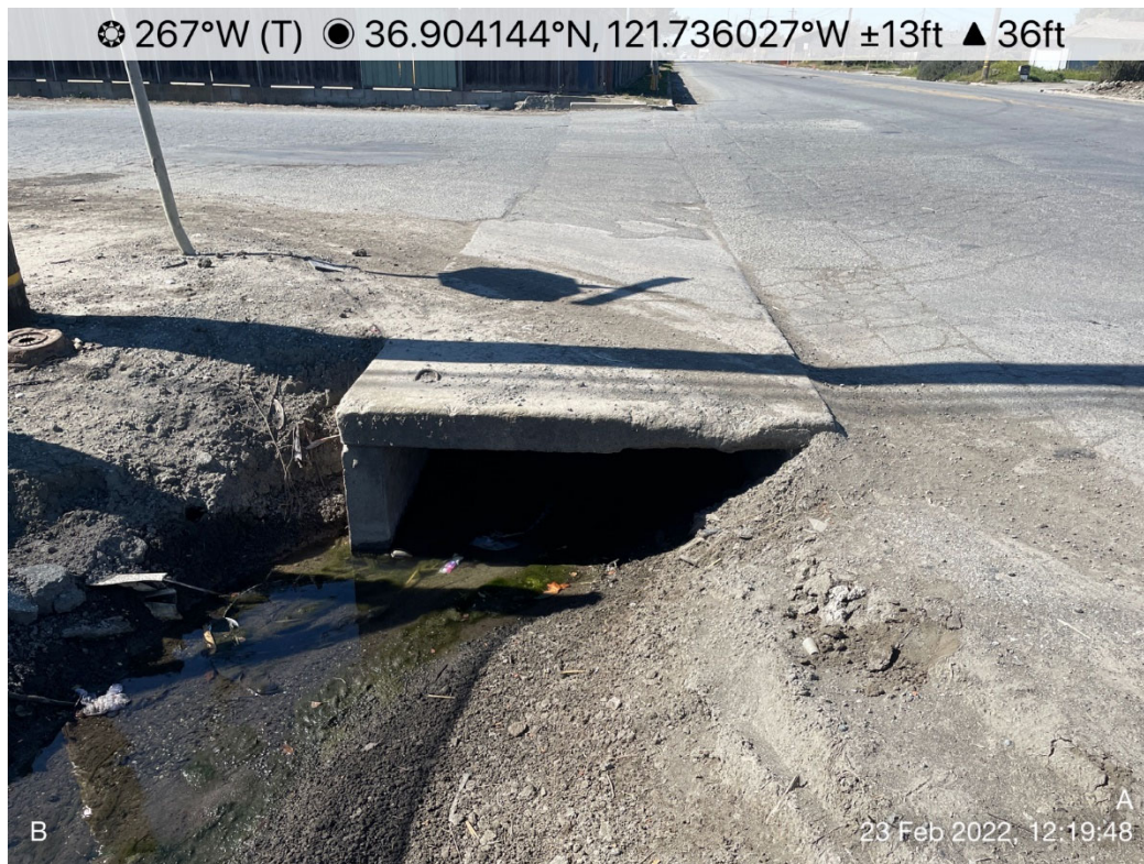
Photo 7. Inlet side of 4.5'W x 1.5'H box culvert crossing Allison Street at San Juan Road. Culvert has a capacity of approximately 22 cfs prior to road overtopping.
