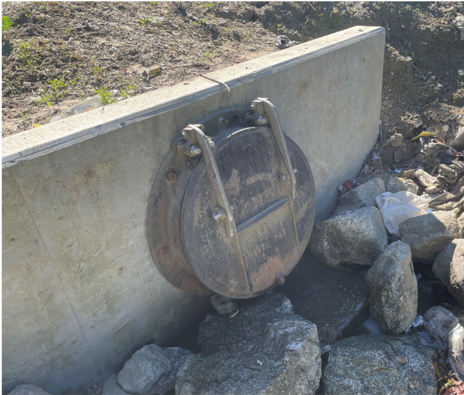
Photo 3. Area B-5 Gravity Outfall near Porter Ave. (30" RCP with flap gate)
