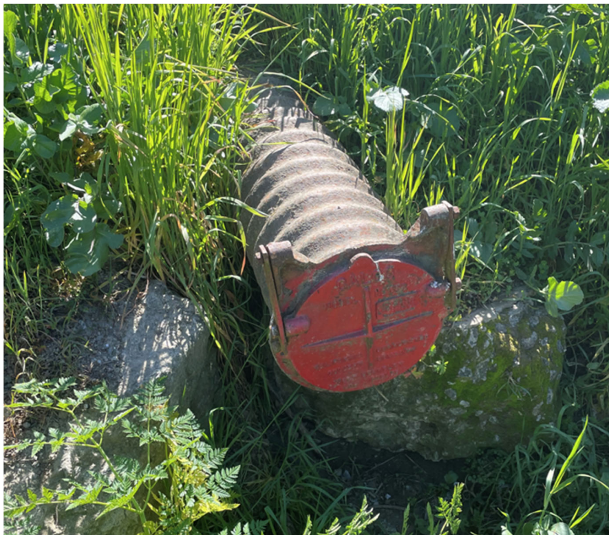
Photo 4. Area B-2 Outfall (12" CMP with flap gate)
