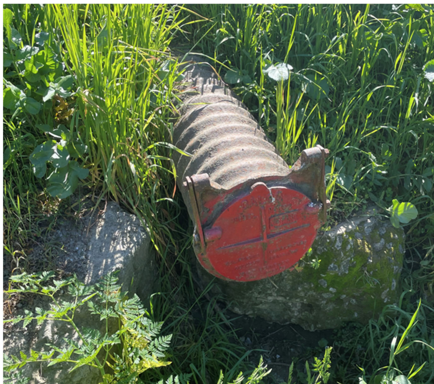
Photo 4. Area B-2 Outfall (12" CMP with flap gate)
