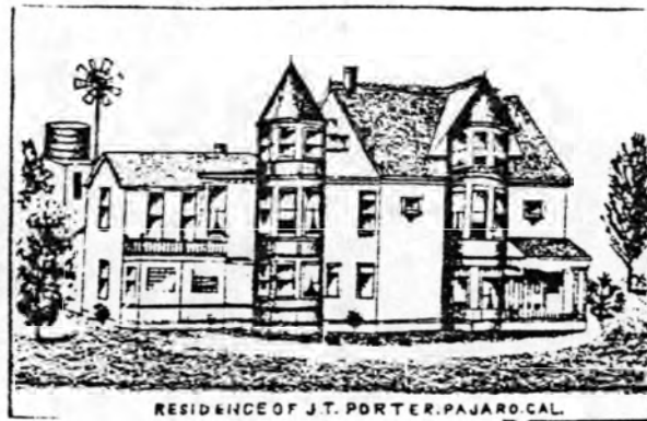
RESIDENCE OF J.T. PORTER, PAJARO, CAL.
