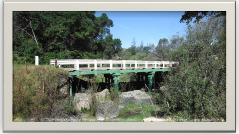
Peach Tree Road Bridge #412 Replacement
