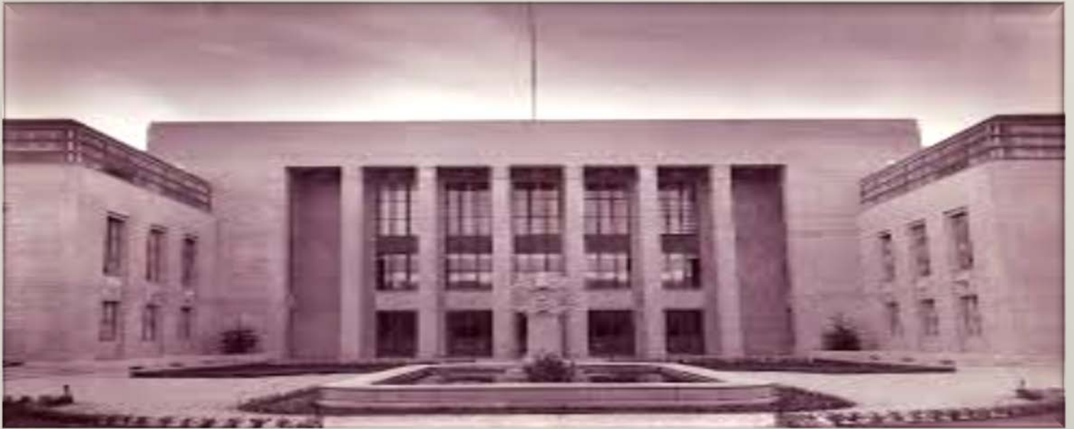
MCGC East & West Wings Renovation
