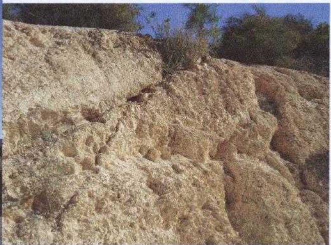
Typical Road Cut (Slope ~ 0.5:1 H:V)
