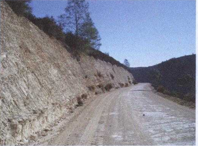
Road Cut View SE Before the Curve (20' Vertical)
