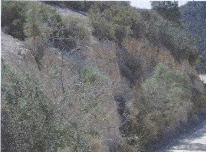
Road Cut Proceeding E from Intersection (7/09)
