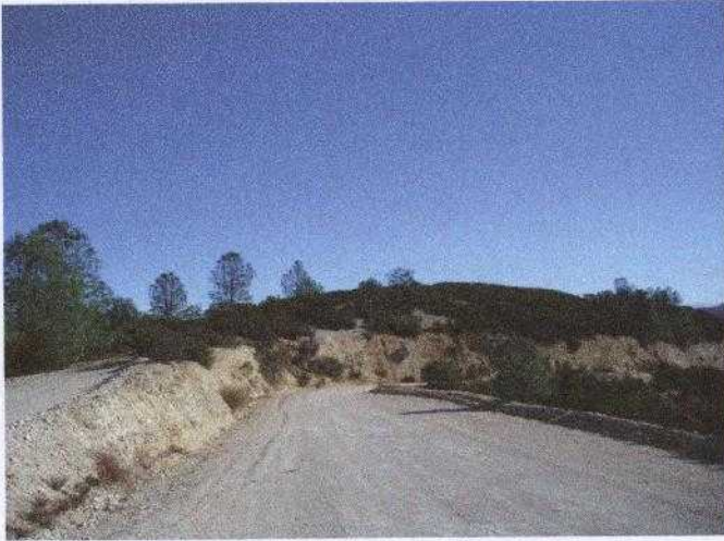
Typical Road Cut (~ 0.5:1)
