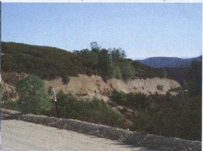
Road Cut W to E (El. 2040 to El. 1960)
