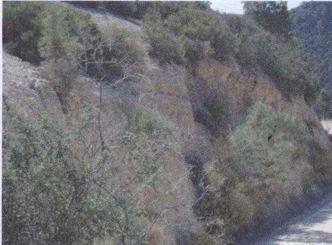
Road Cut Proceeding E from Intersection (7/09)
