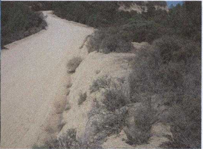
Road Cut starting at Intersection to the East
