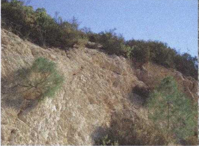
Typical Road Cut (~ 0.5:1)
