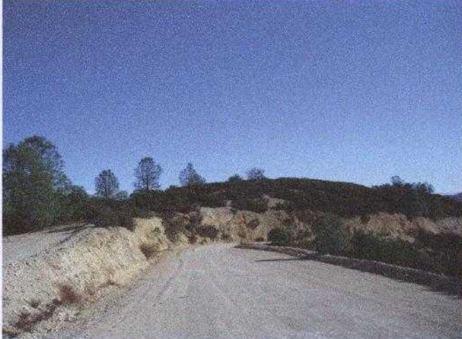
Road Cut Intersection to E (Dec. 2008)
