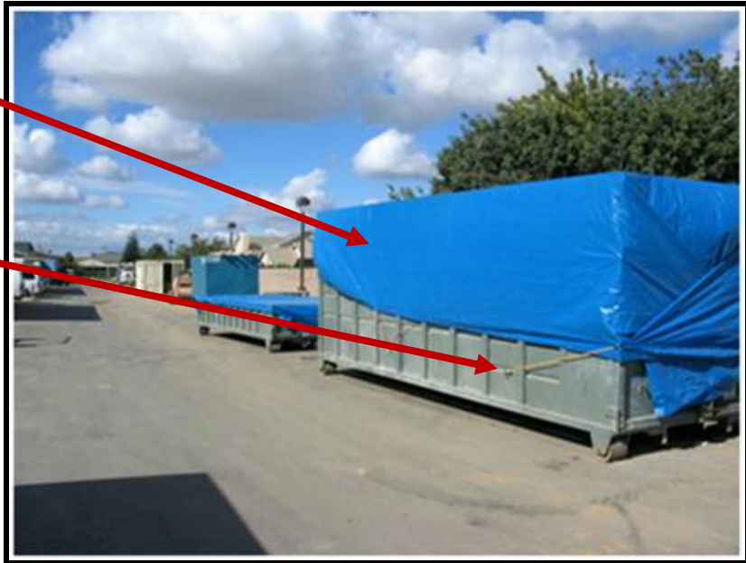
Waste bin with a tarp cover.
