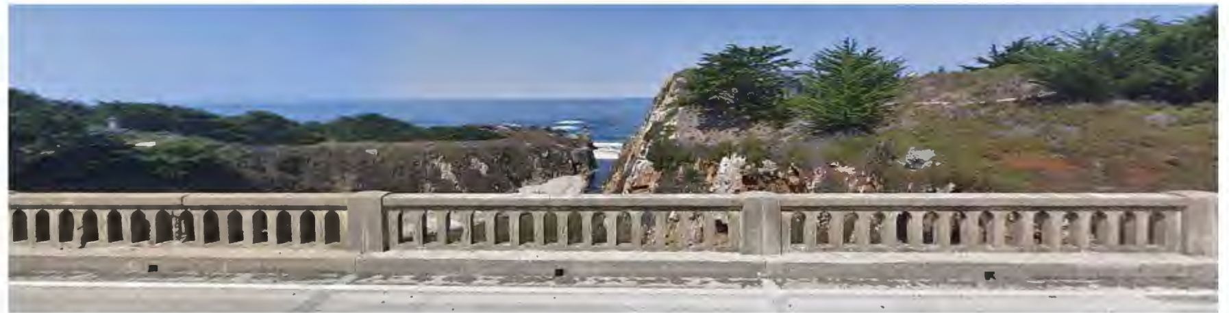
EXISTING ON DECK VIEW
