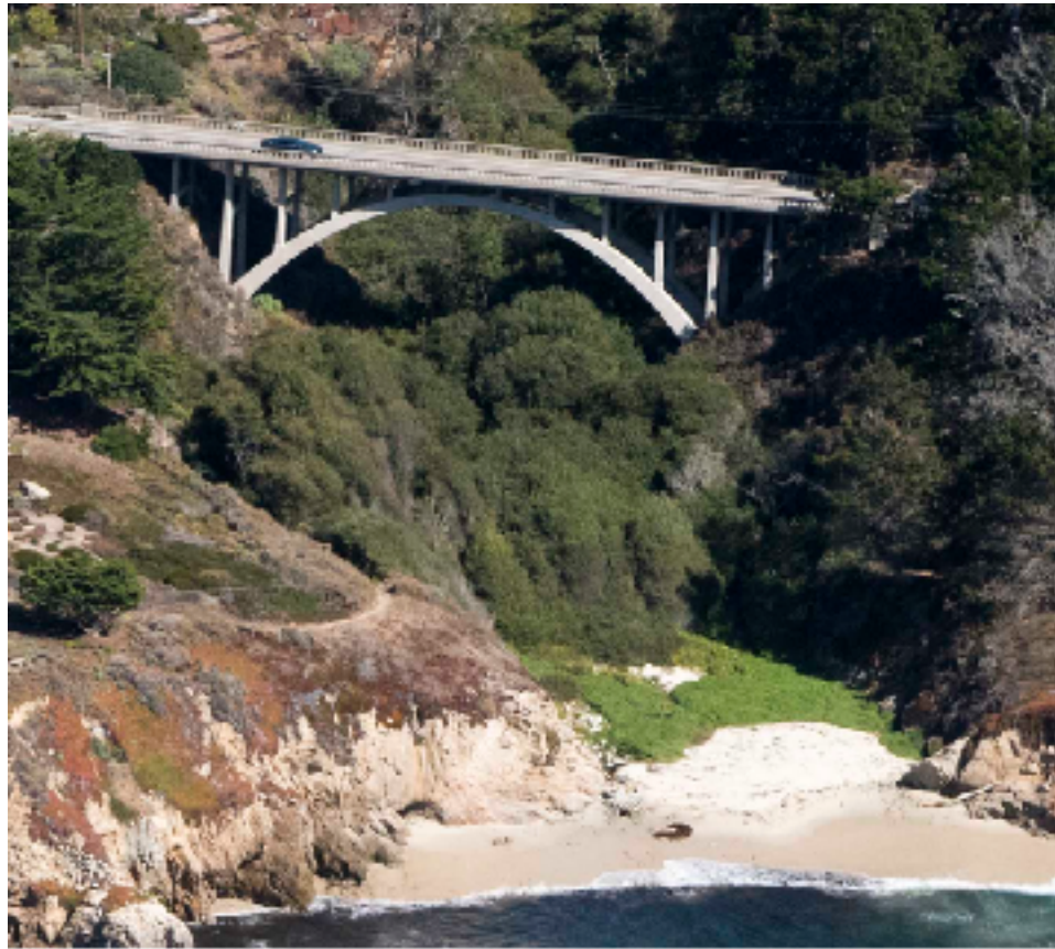
Malpaso Creek Bridge. Photo date: October 2, 2019, excerpt from CCRP Image 201900658.
