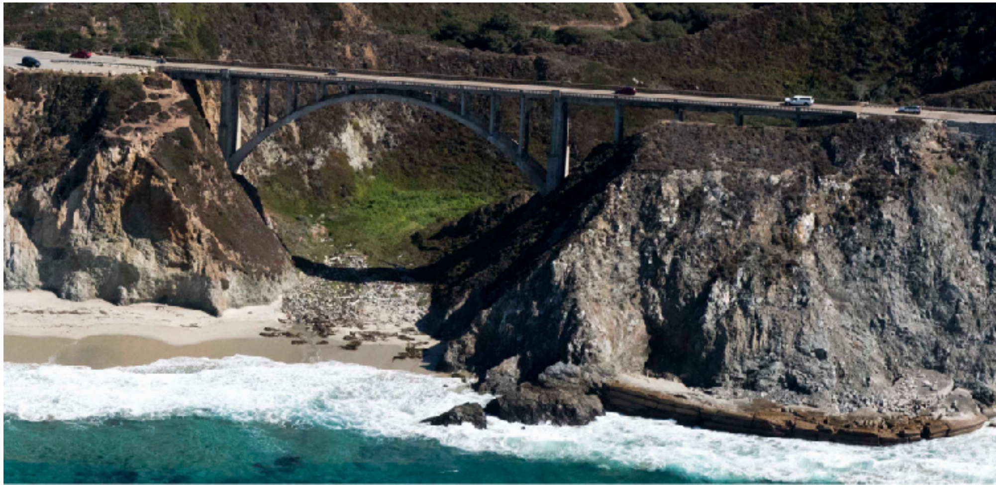
Rocky Creek Bridge. Photo date: October 2, 2019, excerpt from CCRP Image 201900737.
