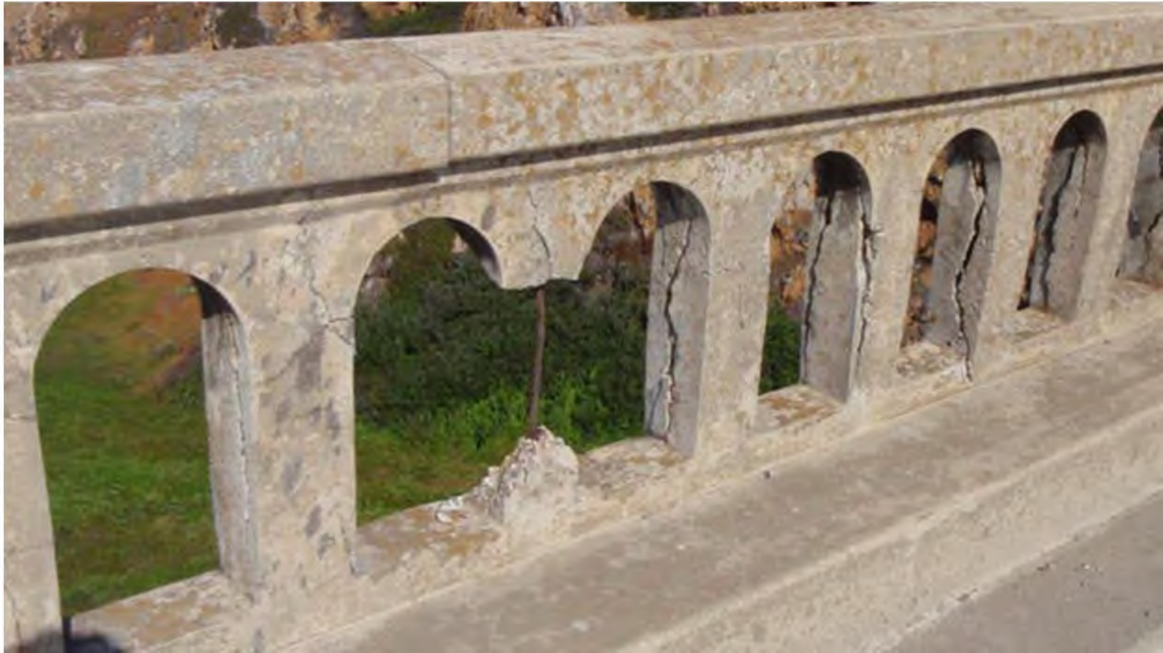
Existing photos of the Garrapata Creek Bridge
