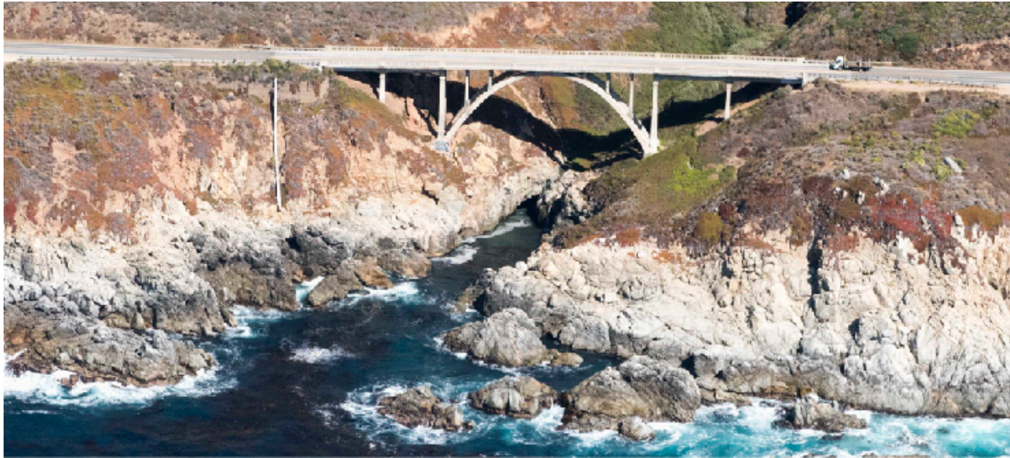
Granite Canyon Bridge. Photo date: October 2, 2019, excerpt from CCRP Image 201900694.
