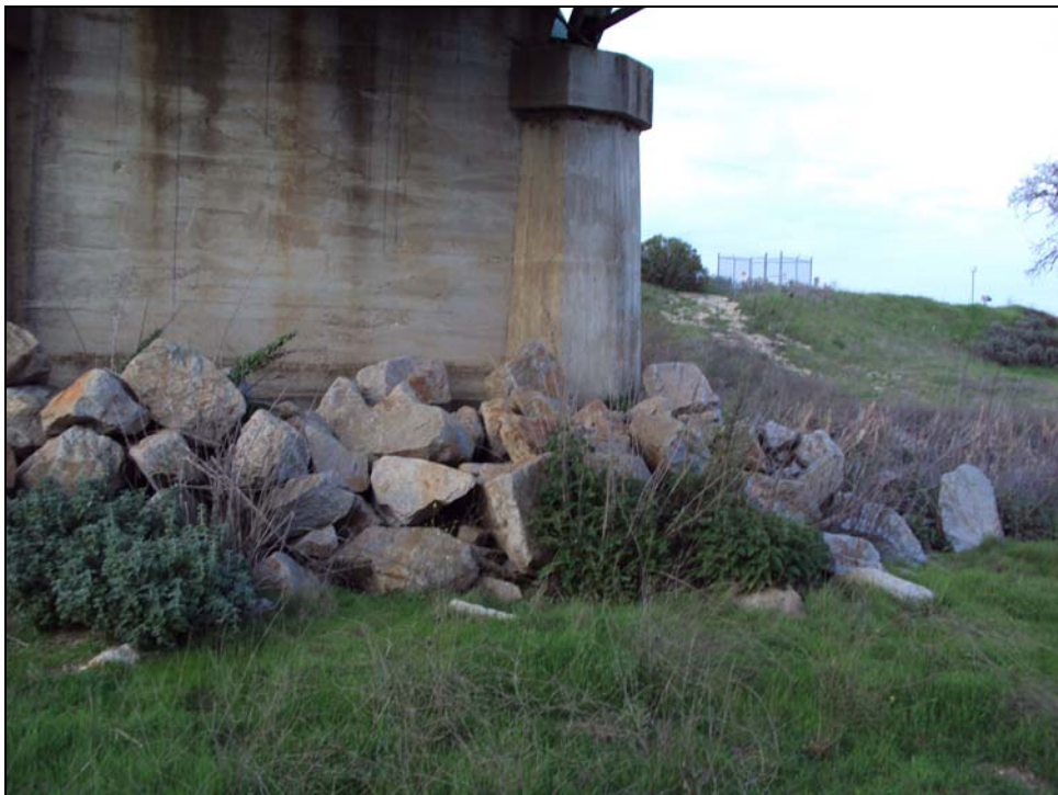
Photo 2. Granite rip-rap around bridge pier.
