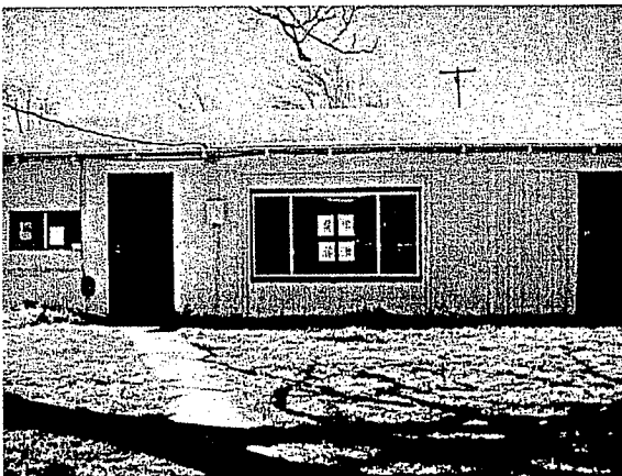
Photo 5: View of the San Lucas County Water District building looking west.
