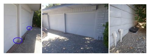
**7. Landscape Design:** Includes improvements to entry gate/fence, wind break fence, bunker, and irrigation and field management, drainage and slope on the property. The inspection report states that surface runoff water be adequately diverted away from the home and lot grading should slope away and fall a minimum of one inch every foot for a distance of six feet around the perimeter of the building.
