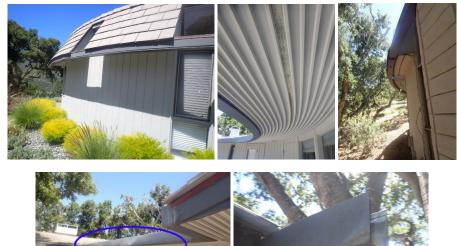
**4. Window and Exterior Door Replacement:** The inspection report states that windows within 24" of ground level should be tempered glass and suggest sealing/ caulking as part of routine maintenance. Areas of calcium water deposit/ moisture damage found on some windows. Replace/restore all windows/ exterior doors throughout home, maintaining original architecture. Replace all window vents and screens, re-paint the interior frame where necessary. Window/ door hardware to be replaced.
