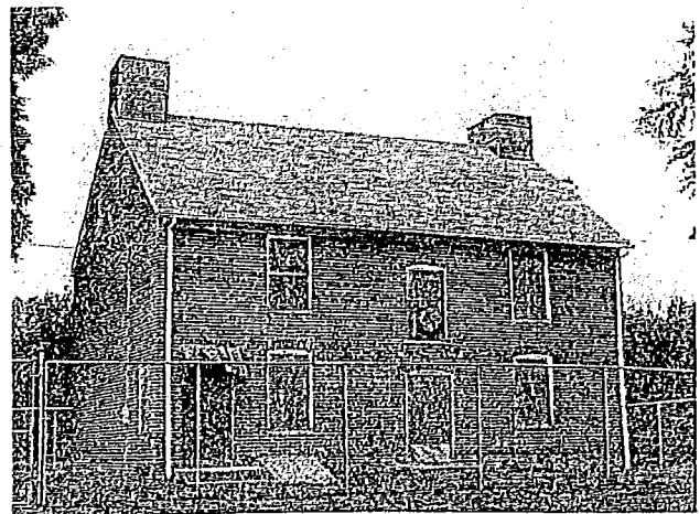
a. A view showing the exterior of the house in its mothballed condition.
