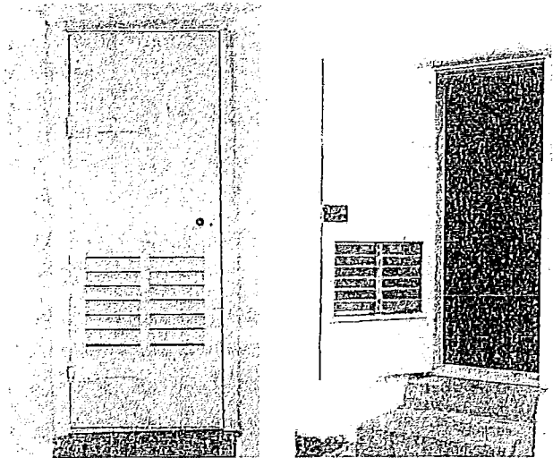
Figure 13. If historic doors would be damaged by adding extra locks, they should be removed and stored and new security doors added. At this lighthouse, the historic door has been replaced with a new door (seen both inside and outside) with an inset vent and new deadbolt locks. The heavy historic hinges have not been damaged. Photo: Williamsport Preservation Training Center, NPS.
