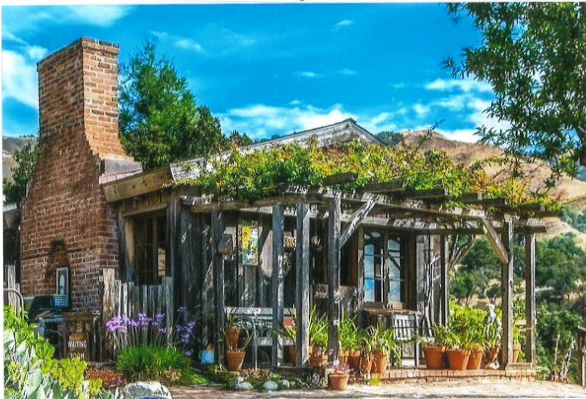
Photo #2. Looking SE at the West facade & North side-elevation, August, 2020, note the undated wood post trellis, wide fascia boards & modified Chimney stack, Robert Carver photo.
