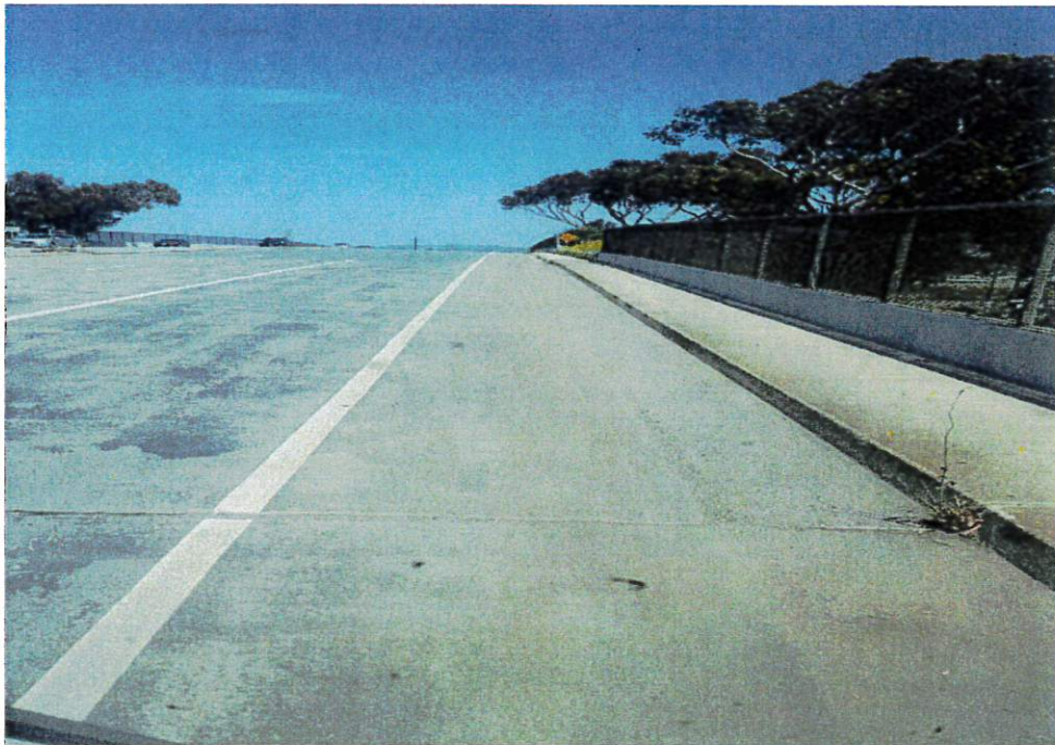
AFTER: Davis Rd. Bridge 5-1-2020 (SAMPLE)
