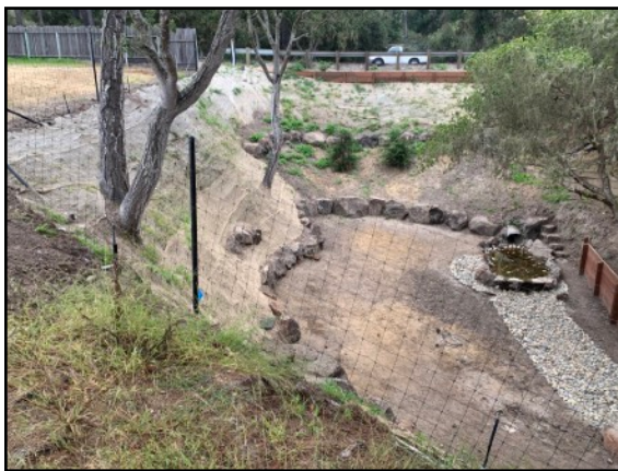
Drainage corridor outfall.
