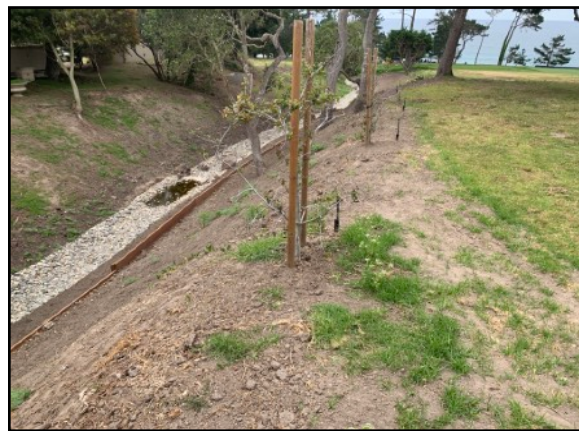
Drainage corridor slope.
