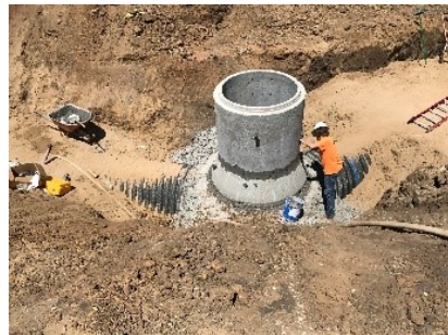
Back-fill of 48" SD manhole.
