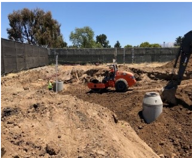
Back-fill of storm drain trench.
