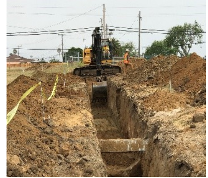
Excavation of gas &amp; water trench.
