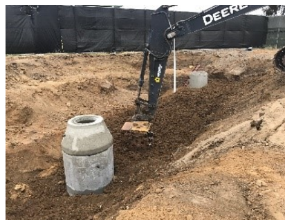
Backfill of storm drain trench.
