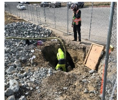
Emergency repair of water leak.
