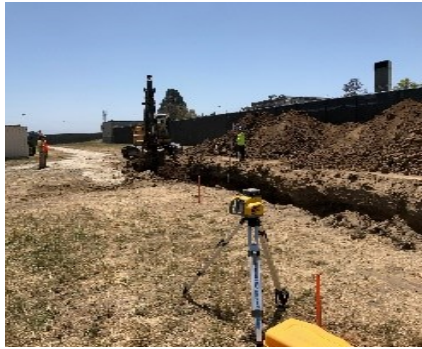
Excavation of 48" storm drain.
