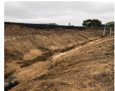
48" storm drain trench partial fill.
