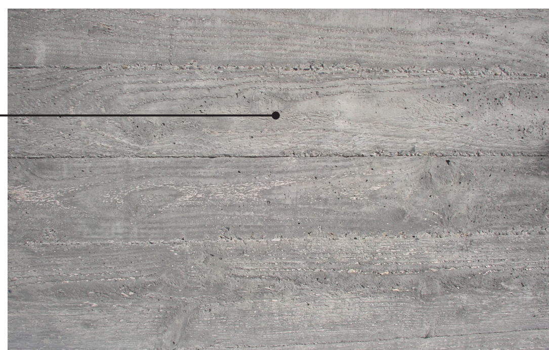
BOARD - FORMED CONCRETE WALLS
