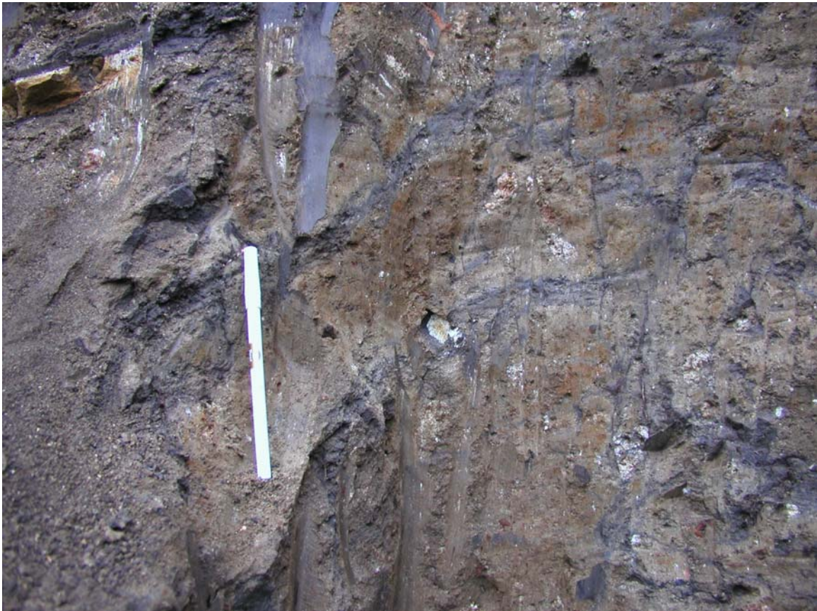
Photograph No. 15: Clay shear surfaces exposed in TP-5, Lot 3.
