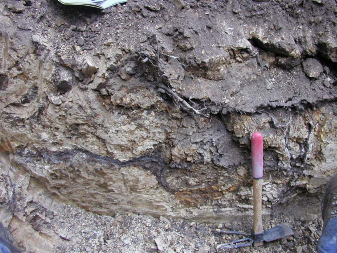
Photograph No. 10: Sheared Monterey Formation siltstone, Test Pit 11, Lot 7. Ground surface at top of photograph.
