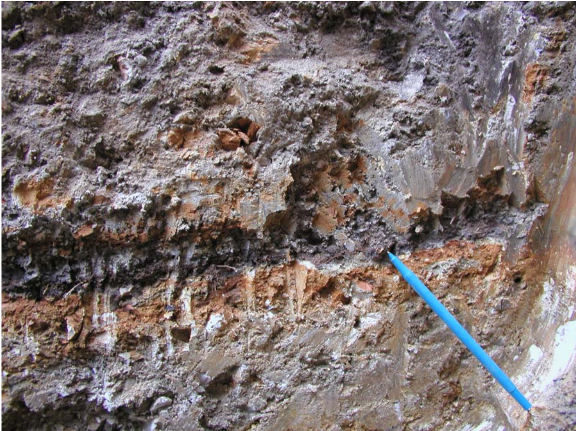
Photograph No. 8: Test pit 13, Lot 9. Head of pen on clay slip surface.
