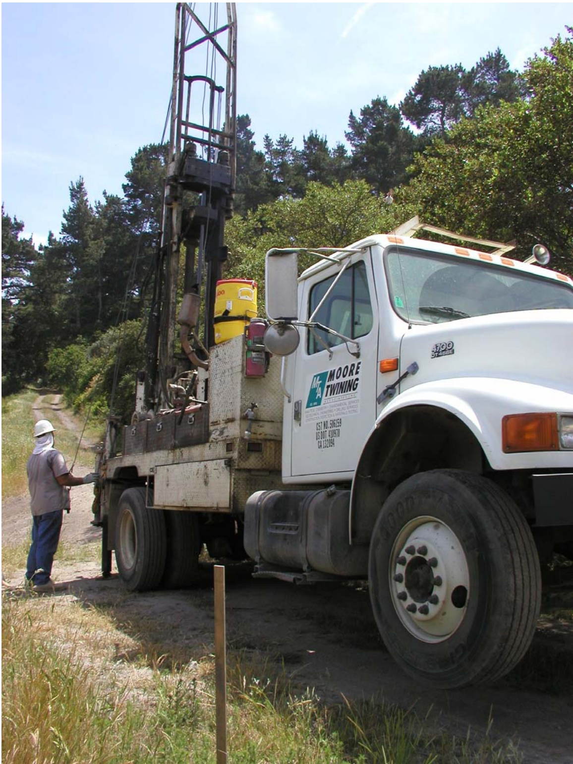
Photograph No. 2: Drilling at test boring B-2.
