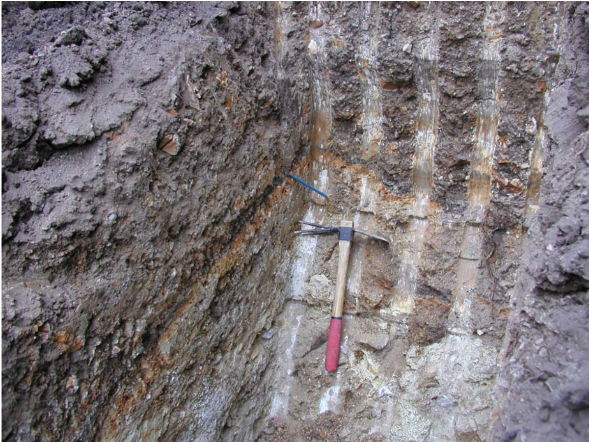
Photograph No. 7: Test pit 13, Lot 9. Pen at clay slip surface.
