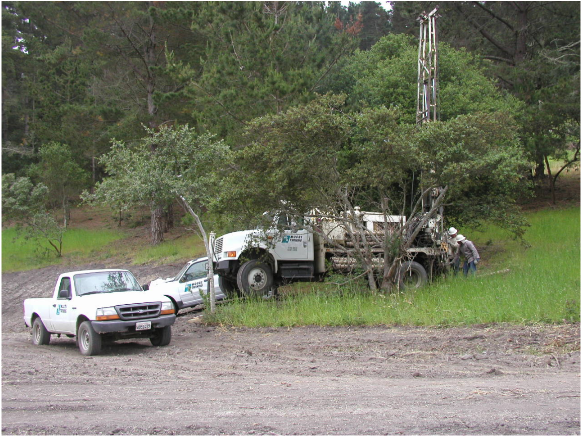
Photograph No. 3: Drilling at test boring B-5, Lot 1.
