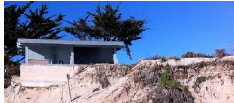
Pictures of Damages in 2023
