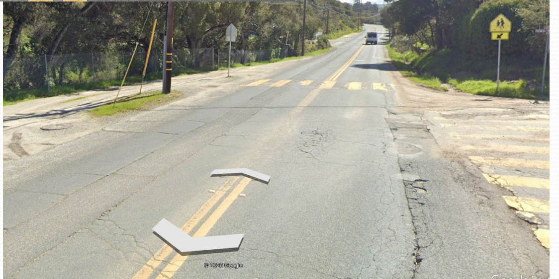
San Benancio Road: Before/After photos
