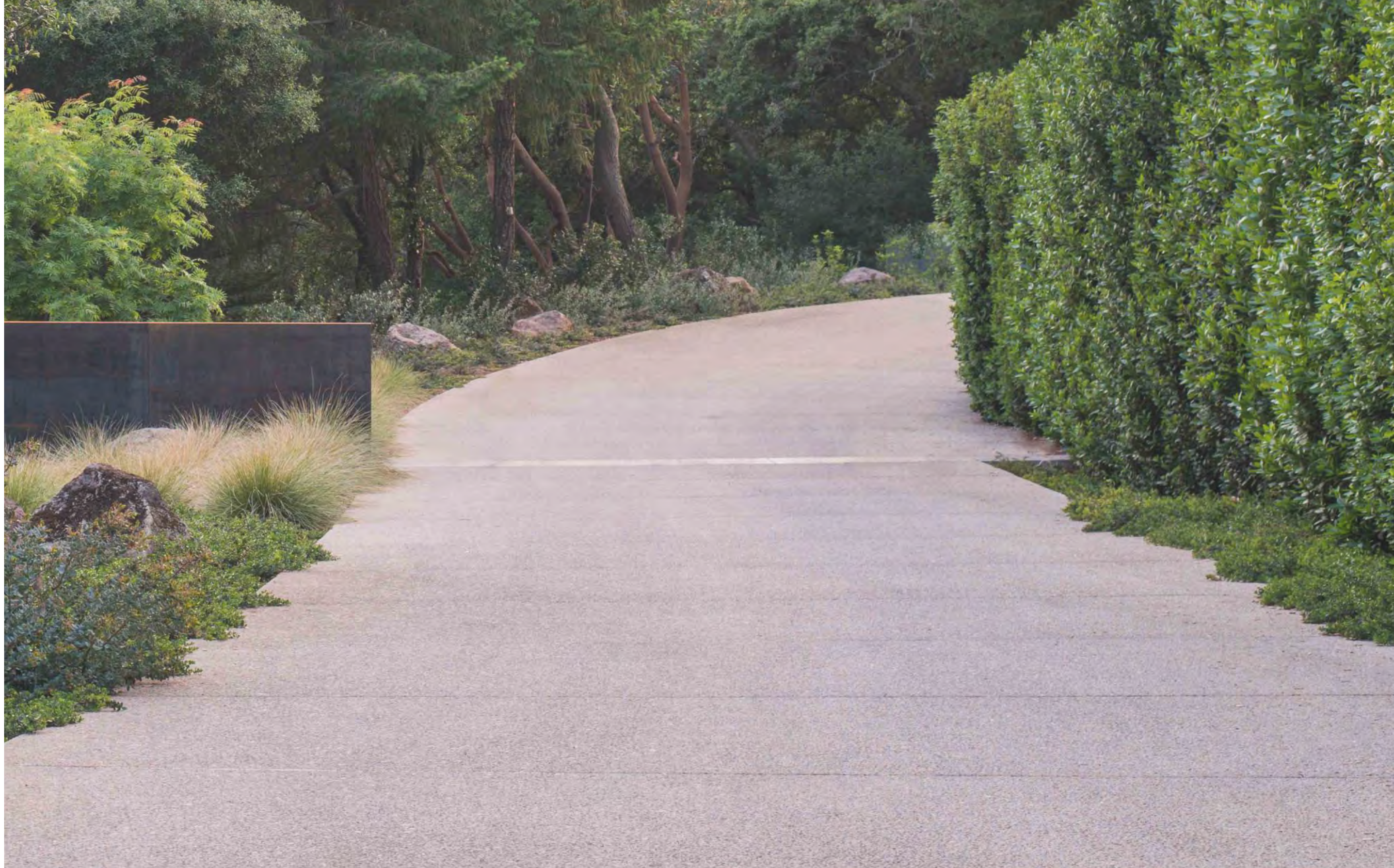
SEEDD AGGREGATE CONCRETE DRIVEWAY
