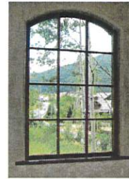
5 WOOD WINDOWS & DOORS
