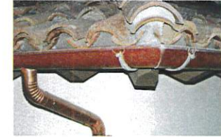
2 COPPER GUTTER & DOWNSPOUT
