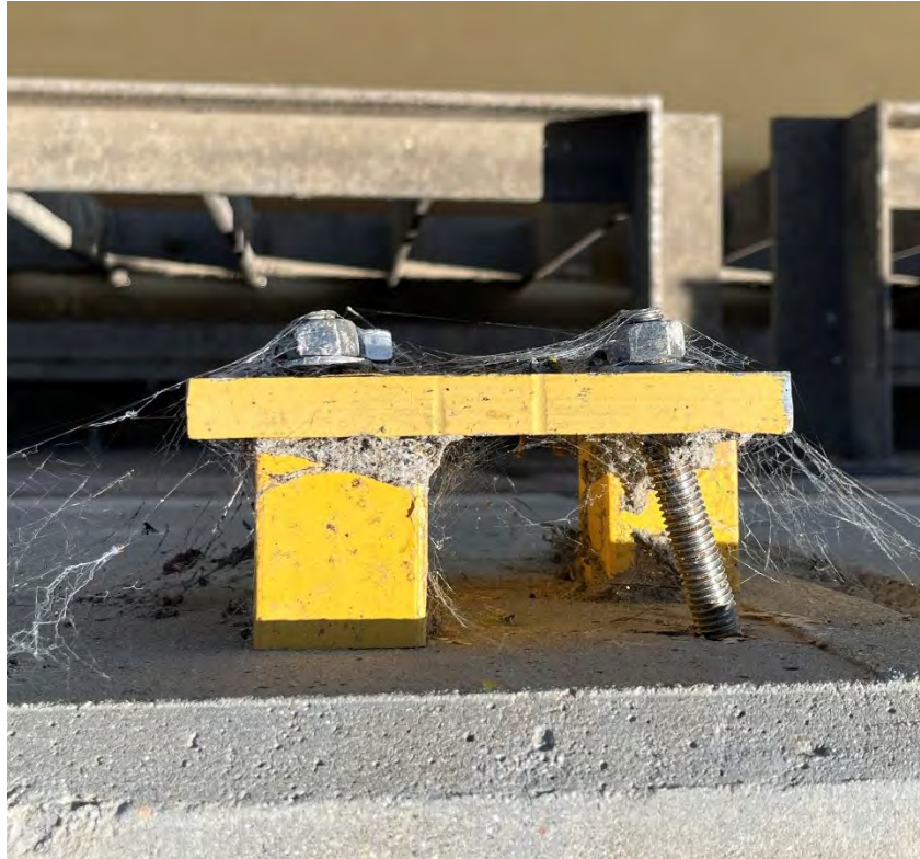
Figure 4: Damaged Rail Support
