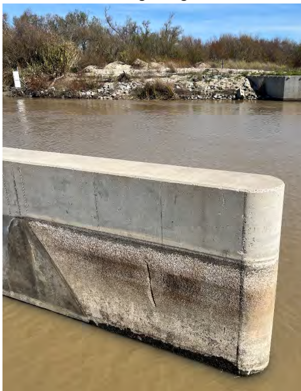
Figure 1: Gash in abutment
