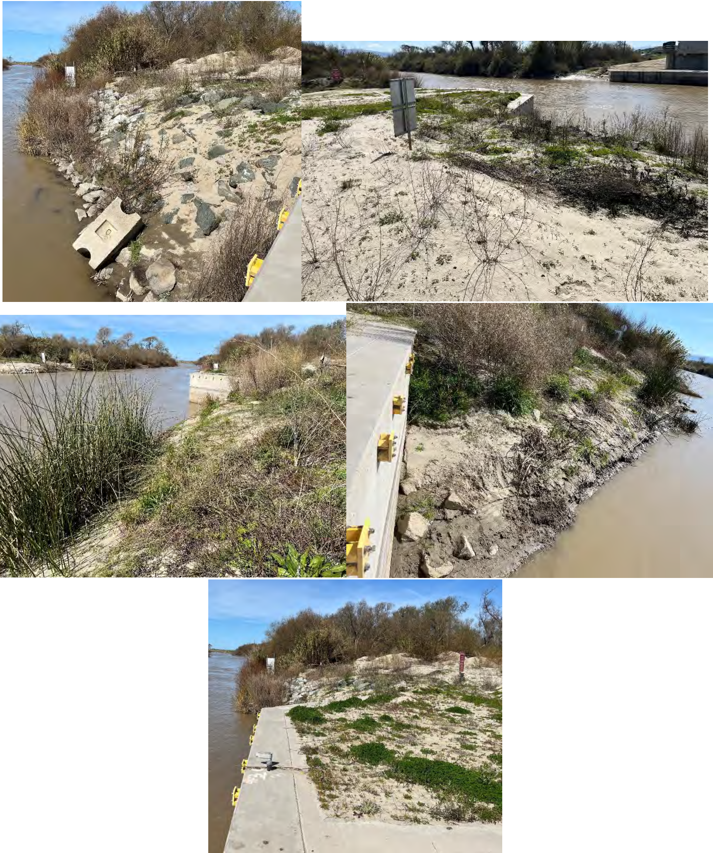
Area 2 RB wing walls: remove silt and replace riprap. Area 14,000 sq ft, volume est. 500 yards (ave depth 1 foot)
