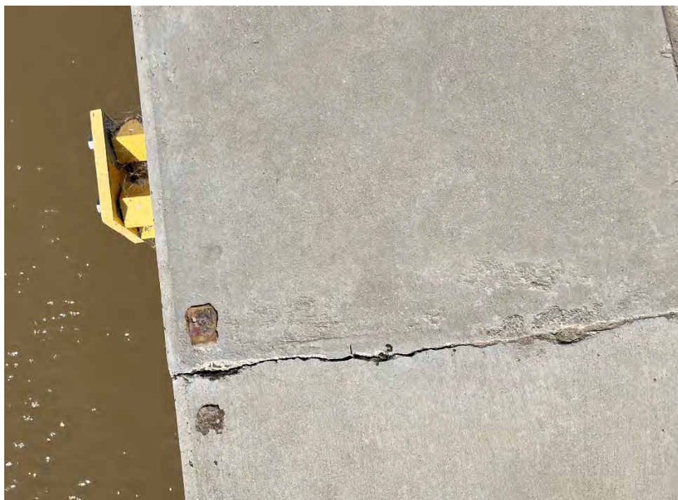
Figure 2: Missing Crack Meter
