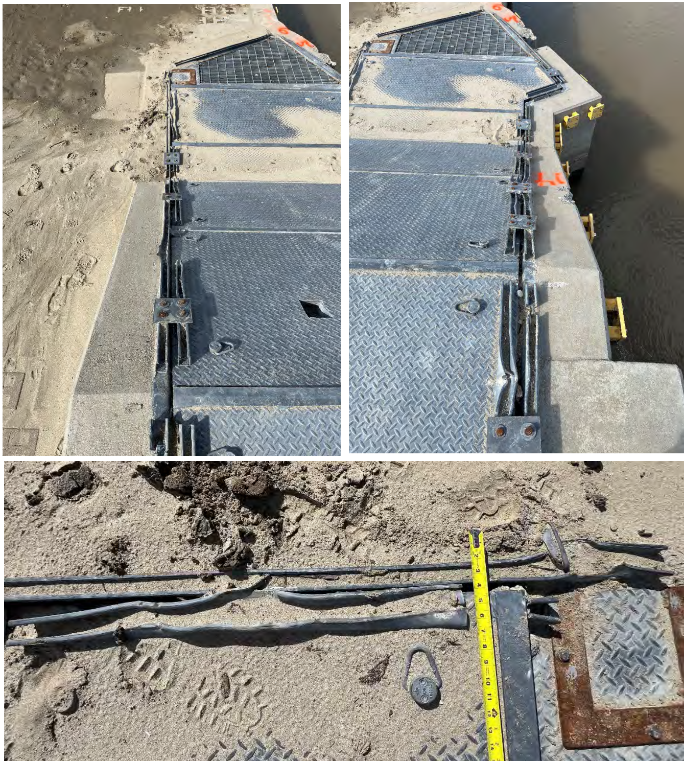
Bent Fish Ladder Top Panels (Three panels damaged)
