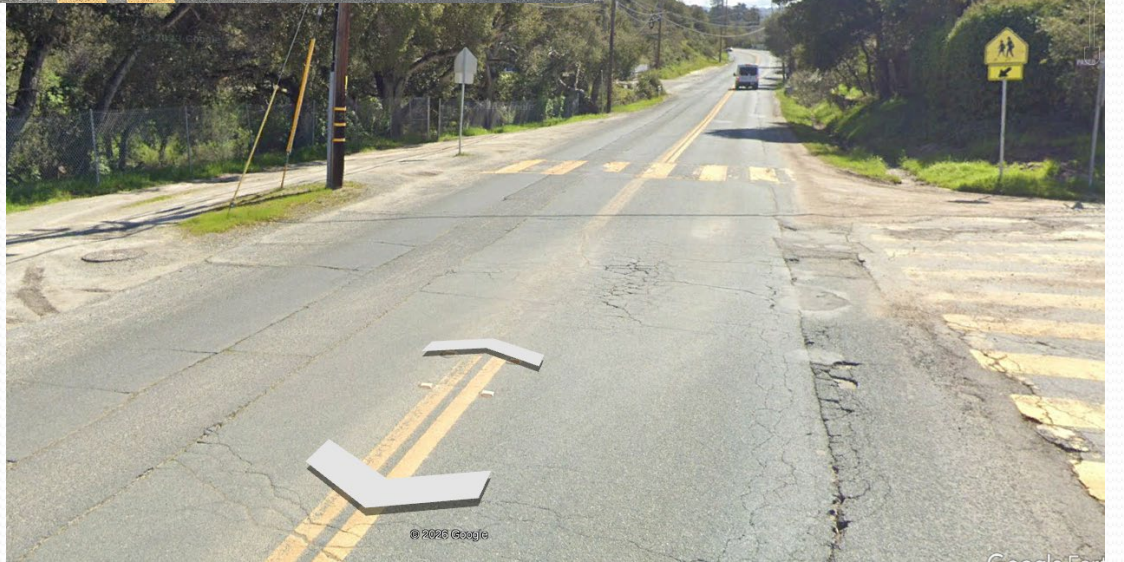
San Benancio Road: Before/After photos
