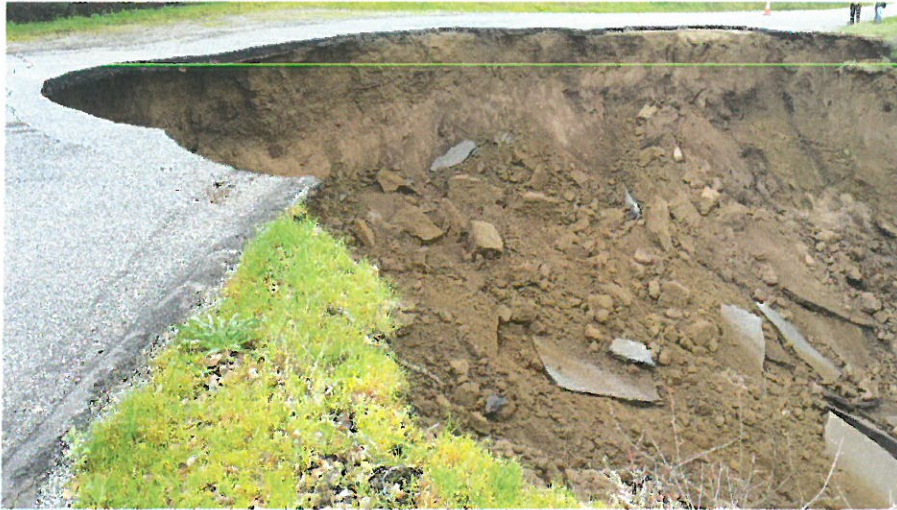
Cachagua Road, 1.5 Miles from Carmel Valley Road
