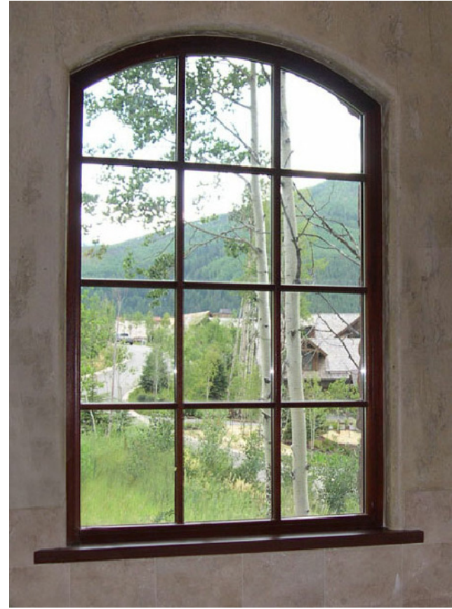
5 WOOD WINDOWS & DOORS
