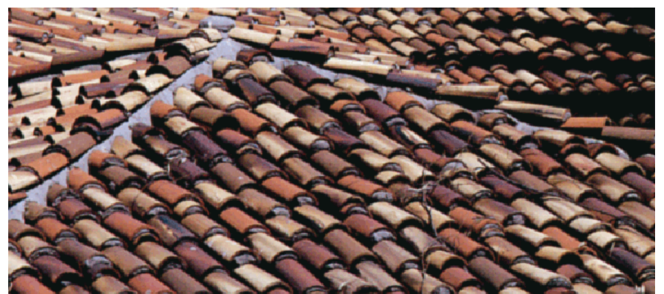
1 CLAY TILE CLAY TILE ROOF
