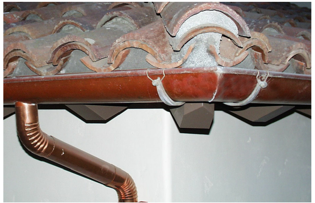
2 COPPER GUTTER & DOWNSPOUT
