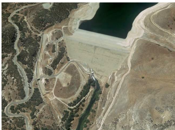
San Antonio Dam and Spillway
