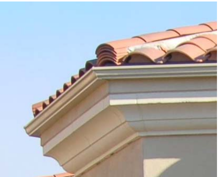
SIMULATED LIMESTONE CORBELS, CROWN MOULDINGS, COLUMNS PLINTH, SILLS, SURROUNDING, ETC SIENNA STONE OR EQUAL
