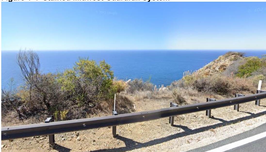
Figure 1-4 Stained Midwest Guardrail System
