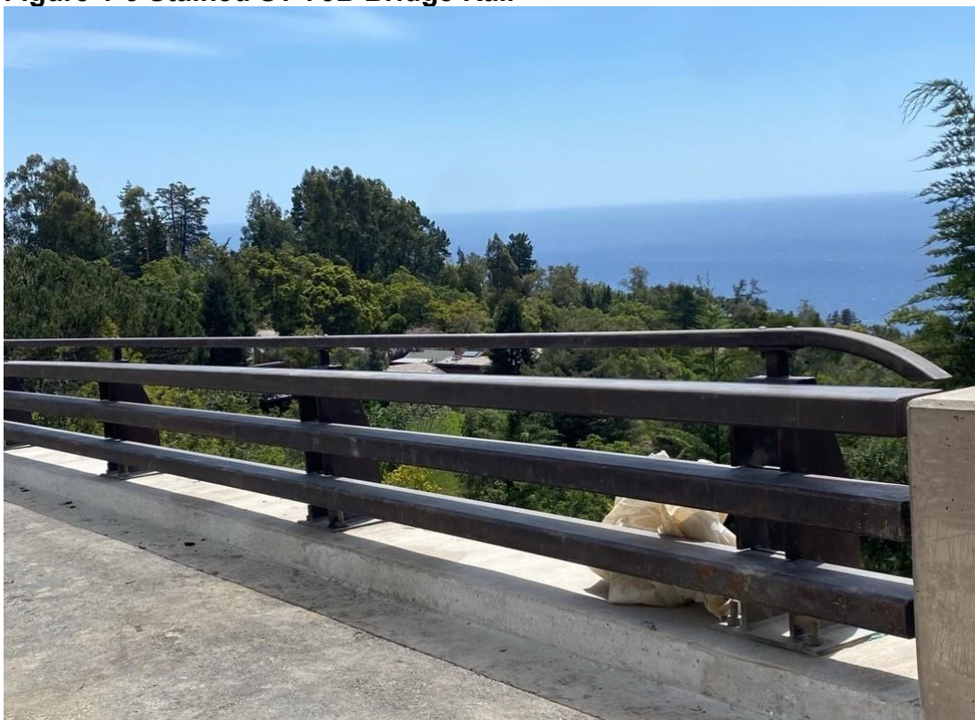
Figure 1-3 Stained ST-75B Bridge Rail
