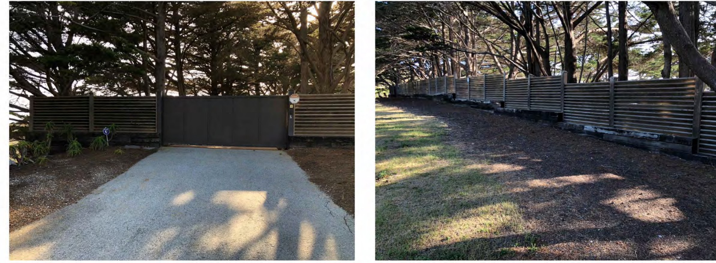
SECONDARY GATE OVERALL FENCE
