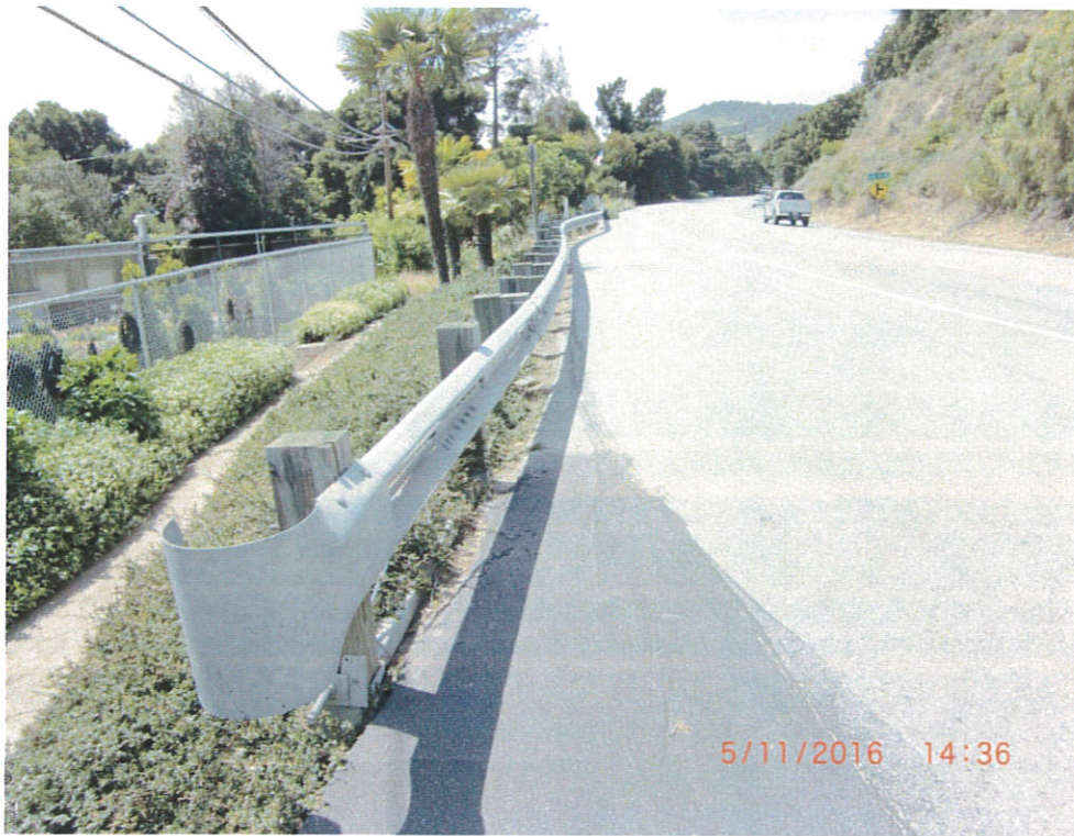
Carmel Valley Road near Loma Del Rey
