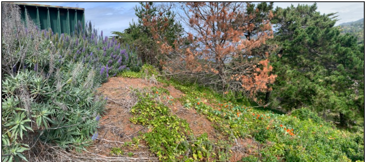
East slope of garage with carpet of invasive cape ivy.
